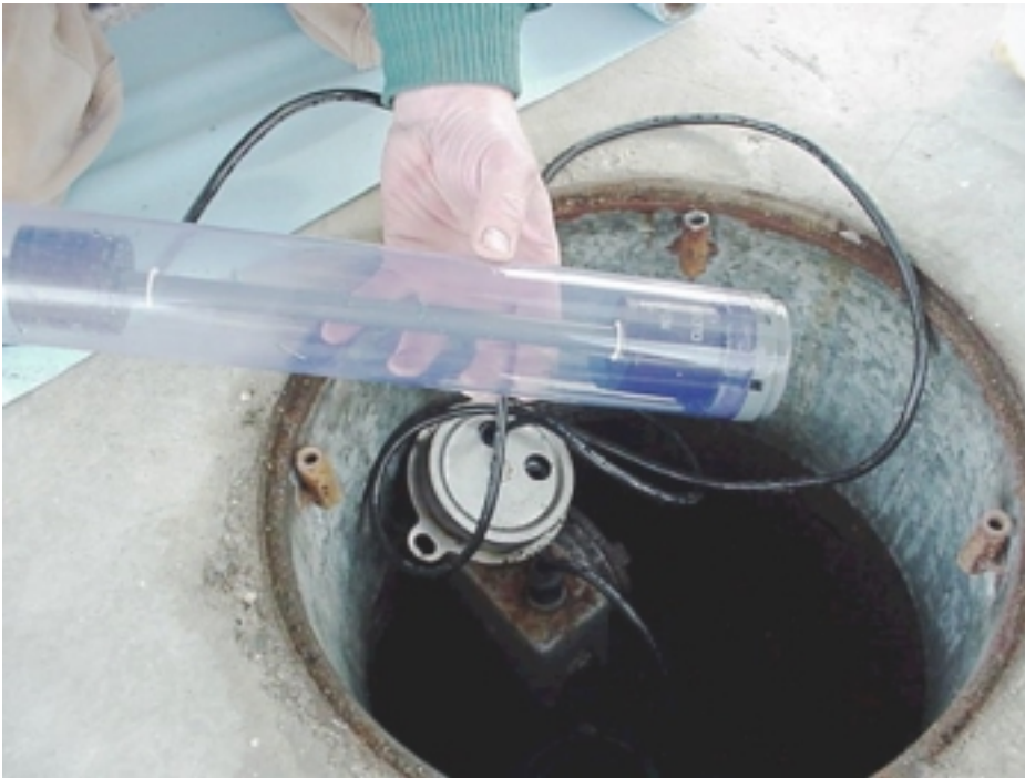
Checking a brine sensor on a double-wall compartment tank in South Central Alaska, 2001.
