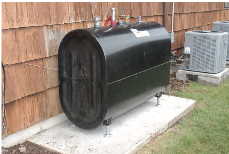
Figure 3-5: Outside above ground tank
