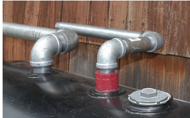
Figure 3-15: Above ground vent pipe/fill and vent cap
