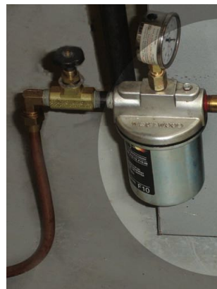
Figure 3-18: Oil filter installed in suction line
