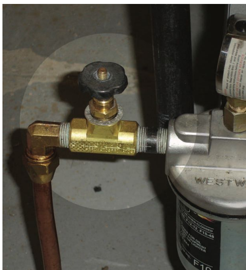
Figure 3-17: Thermal safety shutoff valve
