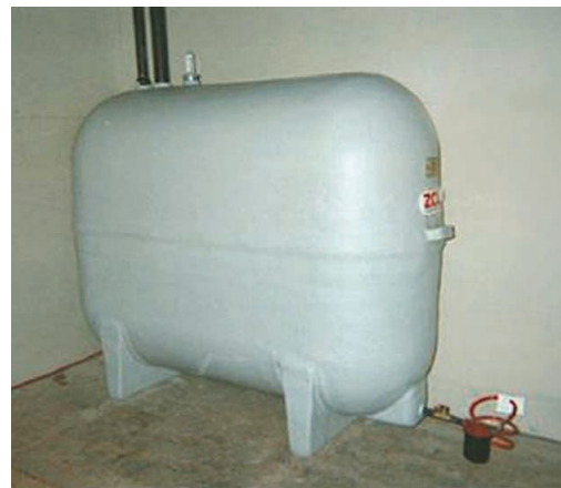
Figure 3-10: Fiberglass tank
