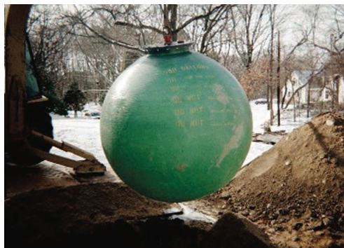
Figure 3-14: Fiberglass (FRP) tank
