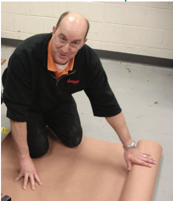
Figure 3-14: Cover work areas
