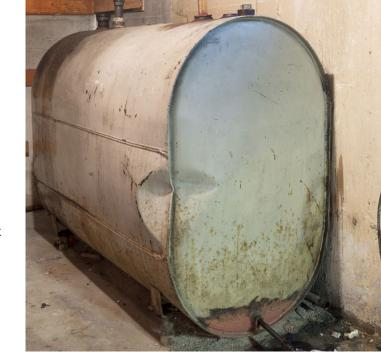
**Closing a Tank:** In the event your heating oil tank is no longer used, the tank must be taken out of service and properly closed. Proper closure for both an AST and UST is defined as emptying the tank and related piping of heating oil. After the oil is drained, the tank must be properly cleaned to remove all vapors and residual oil. Once the AST has been emptied and cleaned and there is no evidence that the tank leaked, the tank is considered closed and can be removed.
