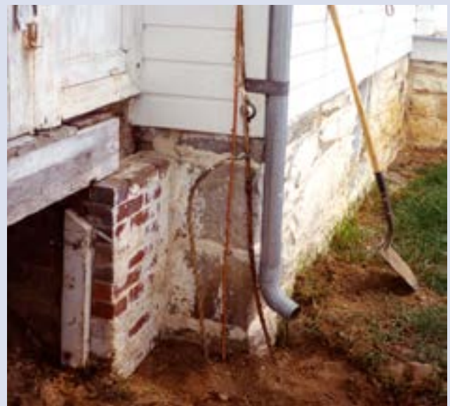
Figure C. The historic down conductor with its original insulator attached to the house just above the stone foundation is still connected to the old ground while bonded to the new conductor and new ground rod.
