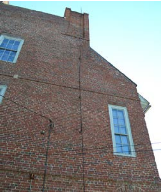
Figure 6. Lightning protection was installed on the Warner House in Portsmouth, New Hampshire, in 1767, purportedly under the personal inspection of Benjamin Franklin. An early system still survives on the building, consisting of a long forged-welded rod of wrought iron which extended up and above the chimney, comprising both the conductor and the air terminal. The conductor was joined to a separate, buried, iron ground rod by a forged hook and eye connector. Photo: Peter Michaud.
