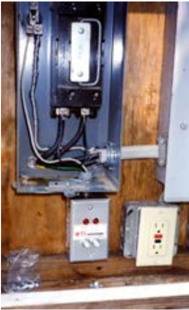
Figure 12. A surge protector covering the electrical lines in a house, barn, or other such structure is relatively inexpensive to have installed. With two or more electrical service boxes, each will need one. The surge protector includes one or more LED lights which indicate whether or not it is properly functioning. In areas of frequent thunderstorms, the unit may need to be replaced after a severe or repeated number of power surges in the line. Photo: Independent Lightning Protection Company.
