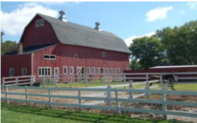
Figure 21. Small air terminals have been used in this more recent installation and have little visual impact. If a partially concealed system was desired, the cable and the mount for two of the air terminals could have been concealed within the ventilators. Photo by author.
