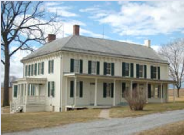
Figure D. Tall lightning rods once again stand out on the Mumma House. These reproduction rods along with retention of the historic down conductors have been incorporated into the modern lightning protection system that was installed. Much smaller, contemporary air terminals located on the roof are barely discernable from below. Photo by author.
