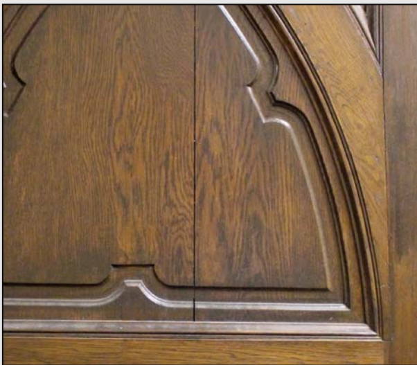
The panel of this old church door has a split. The door is located next to a radiator, exposing the wood to extremely low humidity levels, which more than likely caused the panel to contract and eventually split.
