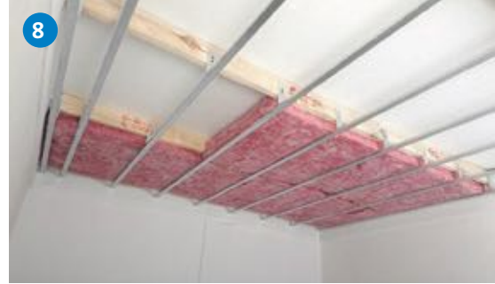
8 After installing the steel branding, install Isovor Aerolite according to SANS 10400-XA for new buildings. (Refer to page 20).
