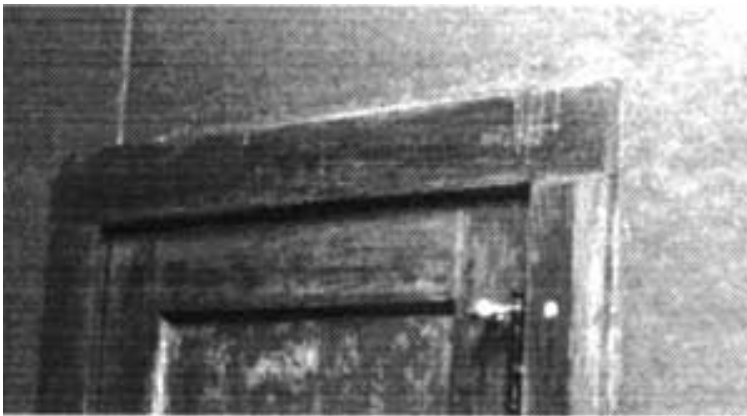
Glaze slopped onto door trim.
