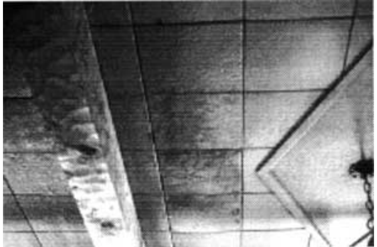
Water damage at the lobby ceiling.
