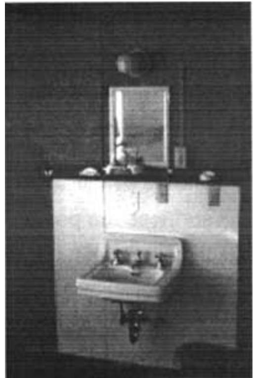
Painted sink surround, 6th floor.
