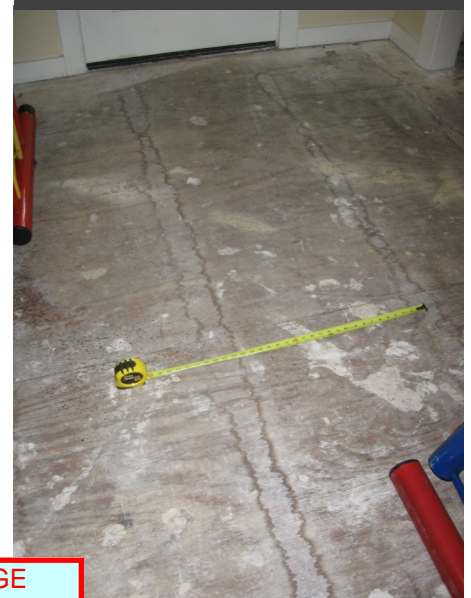
Figure 2. Subfloor with moisture damage in a house with impermeable vinyl flooring (removed) above a vented crawl space
