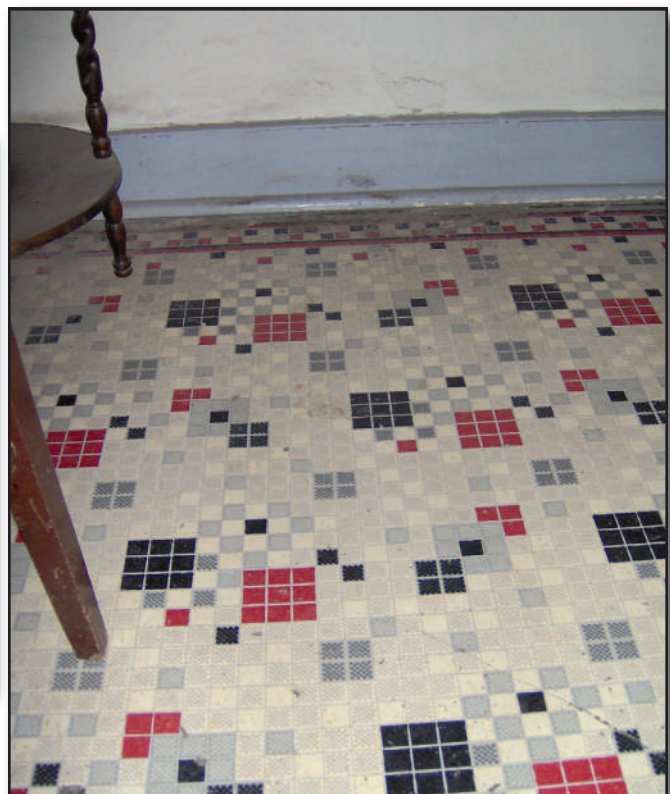
Figure 3—This linoleum flooring is holding up fairly well, but the printed pattern is scratched and worn.
