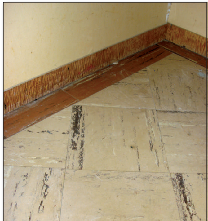
Figure 5—This asphalt tile flooring from 1951 has a darker band of tiles around the edge of the room for contrast and a plywood baseboard that was painted to look like the flooring.
