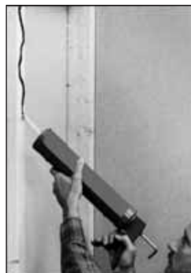
ADHESIVE/NAIL-ON Ideal for prefinished boards.
