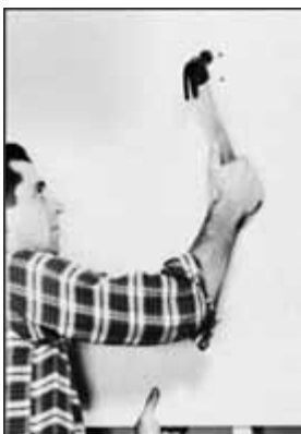
DOUBLE NAILING Minimizes nail-pop.
