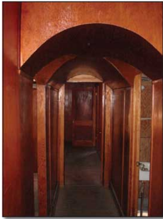
Figure 1—Varnished plywood covers the walls and ceiling of the Rabideau infirmary, which was built in 1935.
