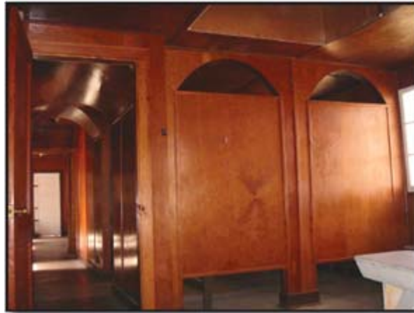
Figure 7—The interior of the infirmary at the Rabideau CCC camp (recently designated as a National Historic Landmark) is finished in varnished plywood, including curved vaults in the hallway and some rooms. Camp Rabideau is part of the Blackduck Ranger District (Chippewa National Forest, Eastern Region).
