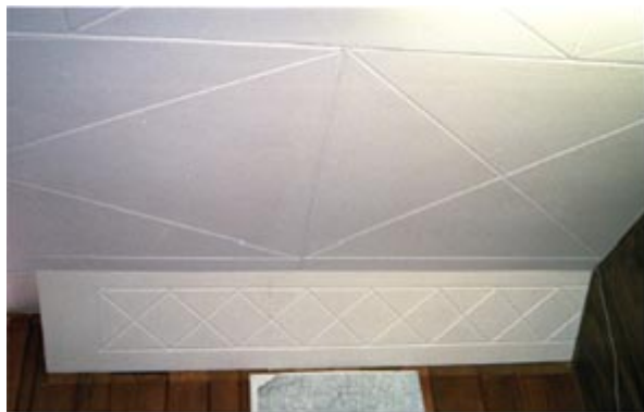
Figure 4—The fiberboard ceiling in the Fenn Ranger Station office (Moose Creek Ranger District, Nez Perce National Forest, Northern Region) has been carved and painted.
