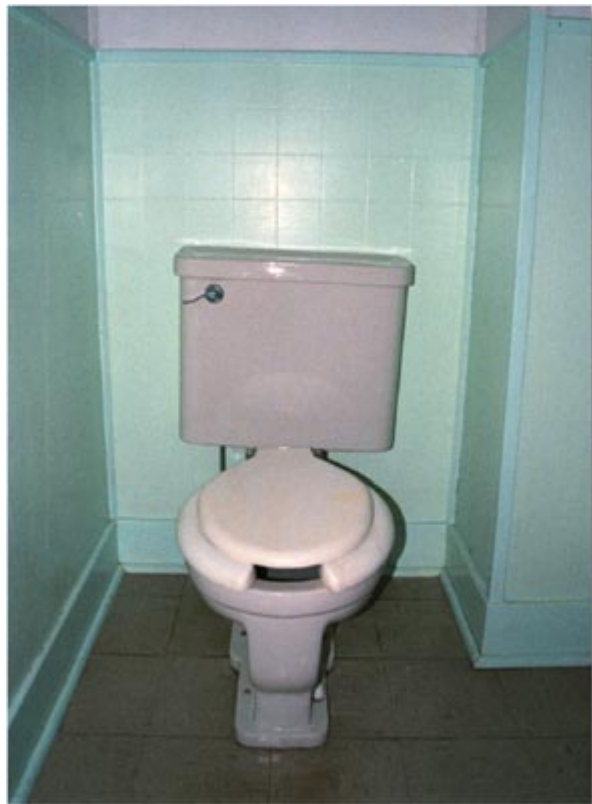
Figure 5—Temprtle, a hardboard product embossed to resemble tile, was used as a water-resistant wainscot in the cook's bathroom at the Fenn Ranger Station.
