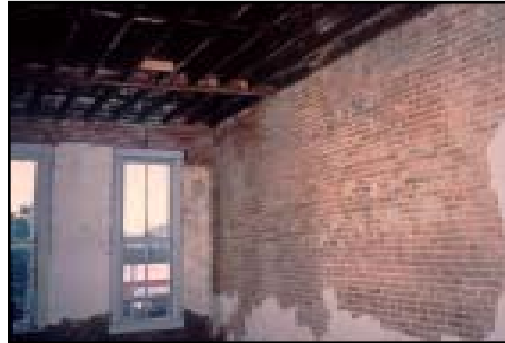
Left and center: Deferred maintenance had resulted in considerable damage to the finished plaster on the upper floors of this small commercial building.
