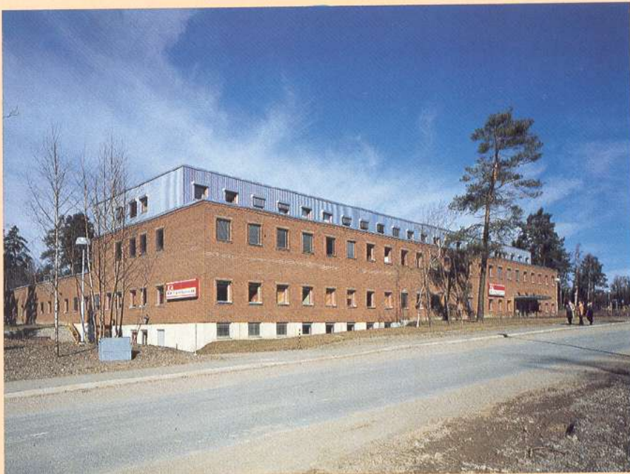
AGA Infrared Systems Headquarters in Danderyd, Sweden.
