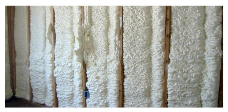
lcynene plastic insulation blown into the walls of a home near Denver. Icynene fills cracks and crevices and adheres to the framing.
