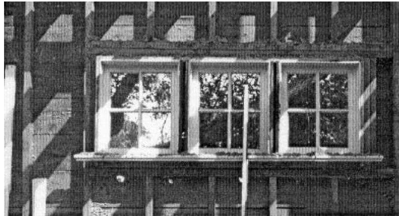
Figure 1: Walls of a wood-frame house built in 1919 at the University of Saskatchewan were retrofitted from the exterior with CFI in 1926 and opened in 1975. Inspection showed no traces of moisture and no visible damage.
