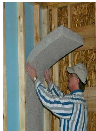
Figure 4: Installation of cellulose batt
