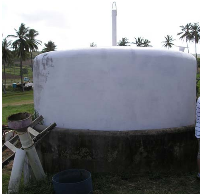
Figure 3.7: Floating drum digester (Richard Hoad Farm)
