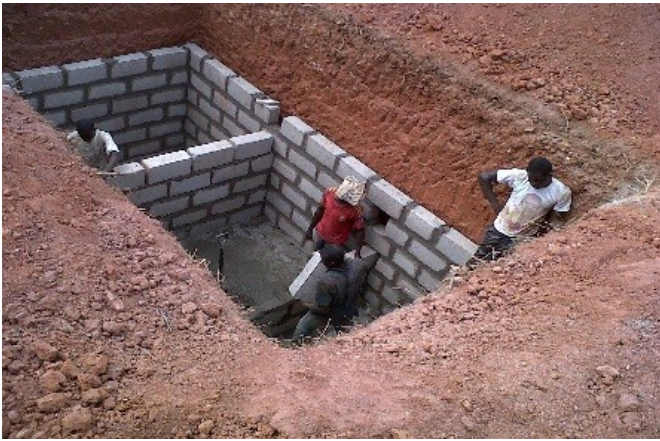
Figure 4. Typical Three-Compartment Septic tank in Ghana
