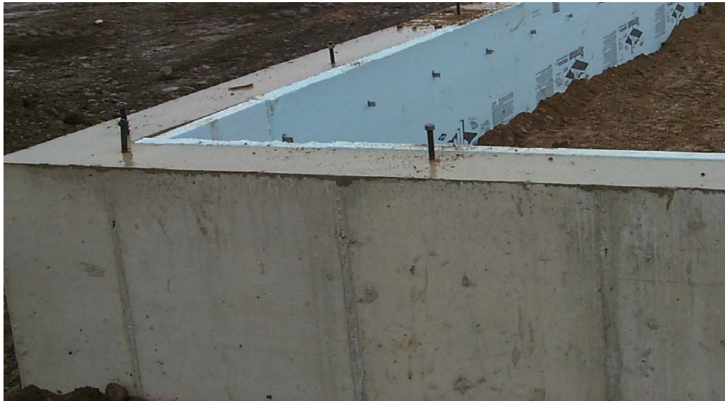
Figure 1: Typical Slab Insulation Installation
