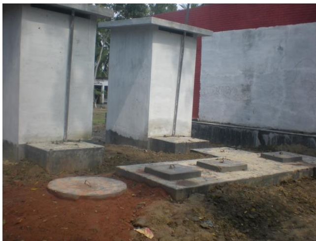
Fig 4.9. A combined septic tank with a common soak pit for two toilets.
