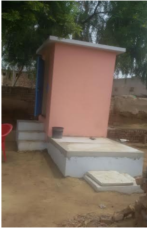
Fig 11. A superstructure with brick cement and RCC roof and plastic door
