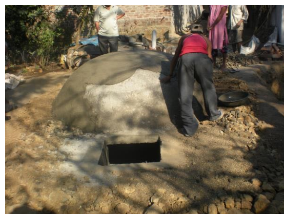
Fig 4.20 A plant under construction (Photo: PK Jha)
