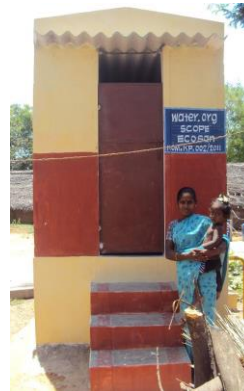
Fig 6. An Ecosan toilet superstructure with brick, cement, and RCC roof and iron door
