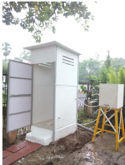
Fig 9 Superstructure of Textile Reinforced Concrete (TRC) with water storage tank found in some parts in Orissa state
