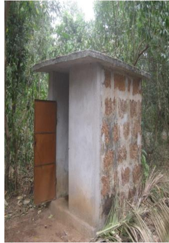
Fig 4 Superstructure with stone wall, RCC roof and iron sheet door
