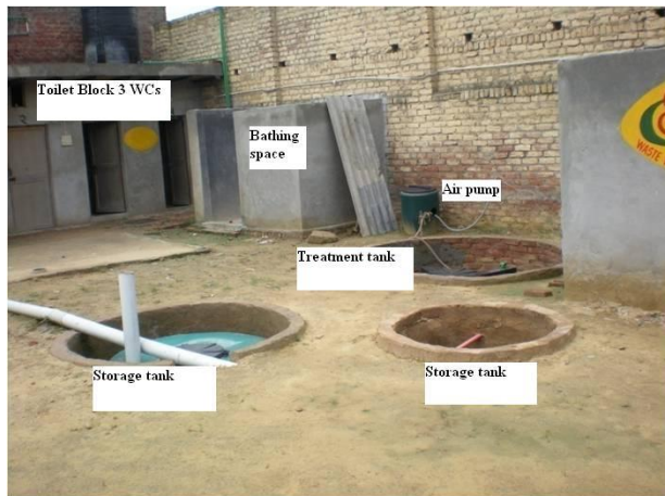
Fig. 4.35 LDDPE made settling –contact aeration system Fig. 4.36 Coirs used as growth medium
