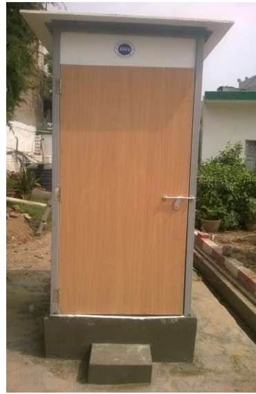
Fig 8 Superstructure with precast ferro- cement slabs
