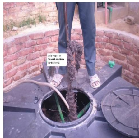
Fig. 4.35 LDDPE made settling –contact aeration system Fig. 4.36 Coirs used as growth medium
