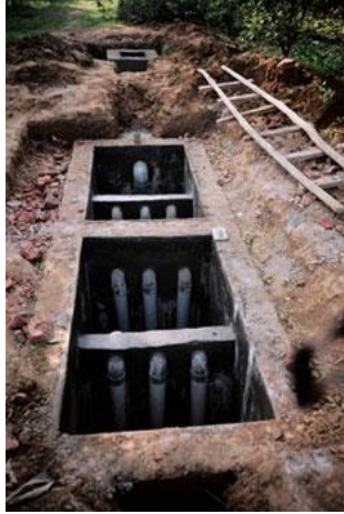
Fig. 4.24: An ABR under construction Source. DEWATS guidelines
