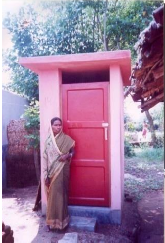
Fig 3 Superstructure with brick, cement and RCC roof and iron sheet door
