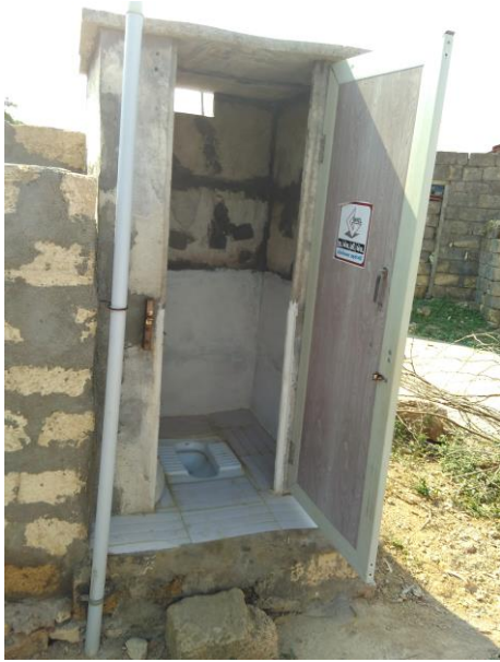
Fig. 7 Superstructure with precast ferro- cement slabs and wooden door used in Junagadh area in Gujarat
