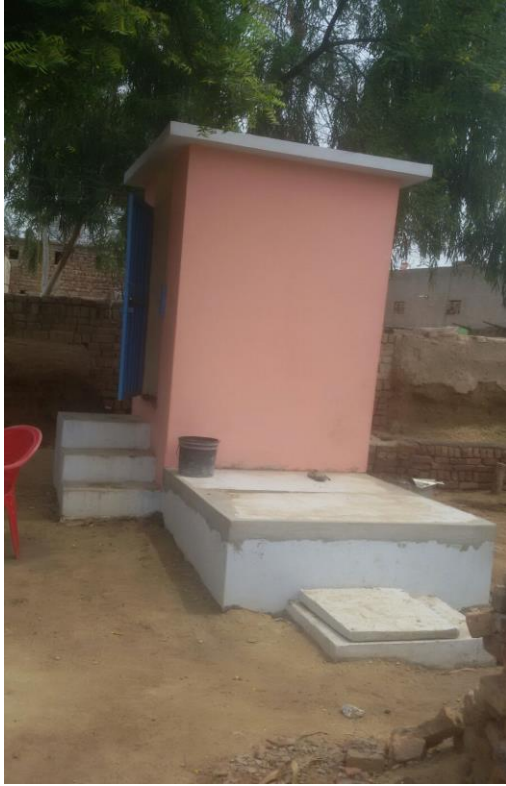
Fig.4.28, Toilet with ABR technology for water logged area Fig. 4.29 Toilet with ABR technology for water logged area
