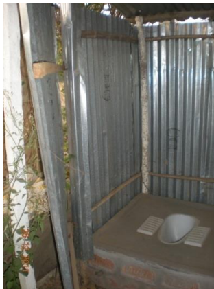
Fig 5 Superstructure with G.I. sheet
