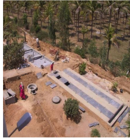
Fig 4.25 An ABR after completion
