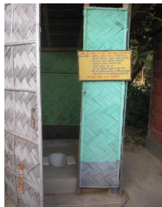
Fig 2 Superstructure with thatch.
