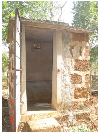
Fig 10. Superstructure with laterite and iron sheet gate
