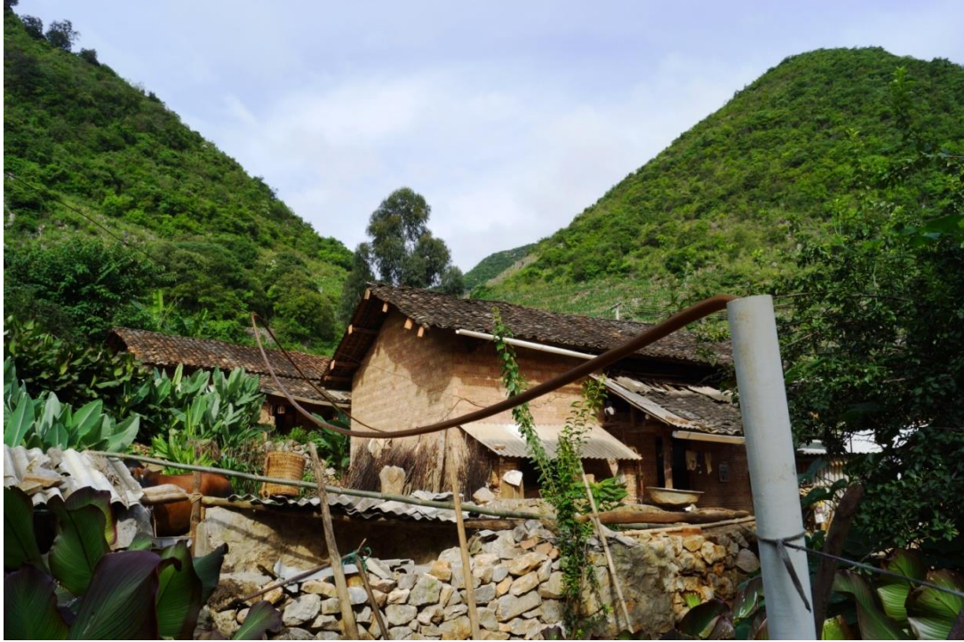
Jiudai Yakou village's electricity transmission lines
