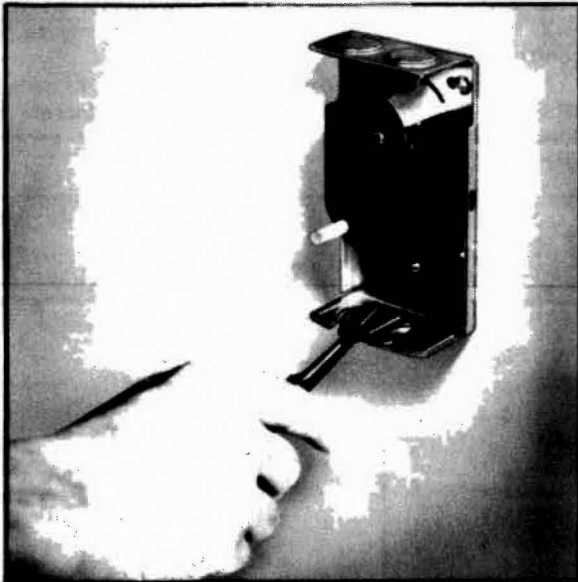
FIG. 6—REMOVING SLOTTED KNOCKOUTS.
