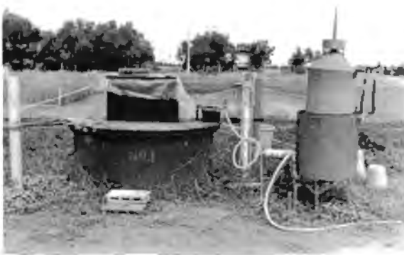
Fig. 6. Ferrocement biogas digester in operation.
