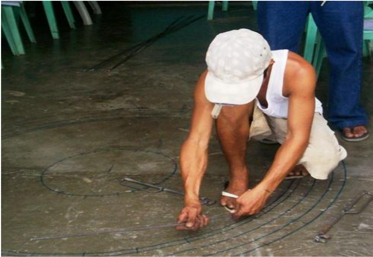
Laying the Patterns
