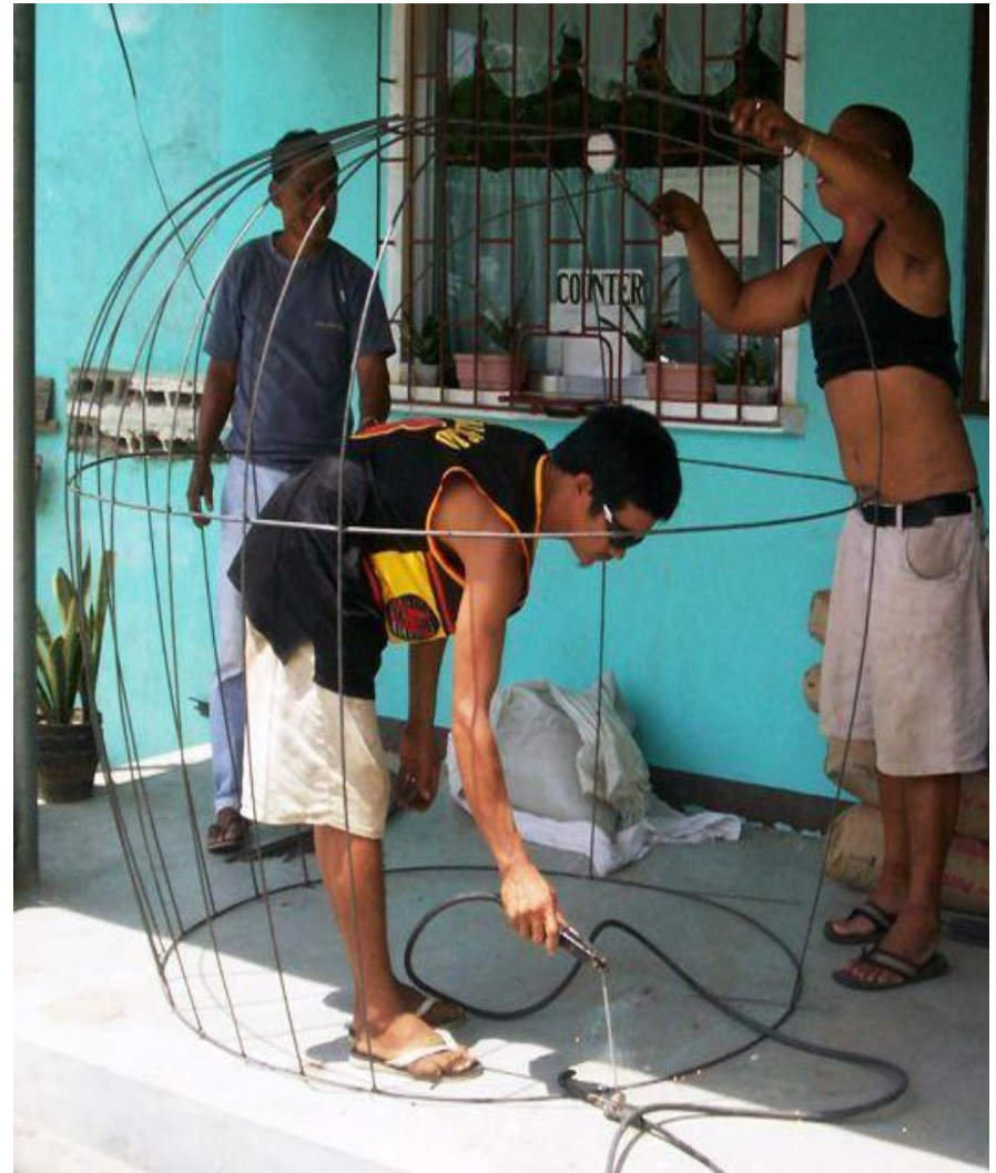
Digester mold welding
