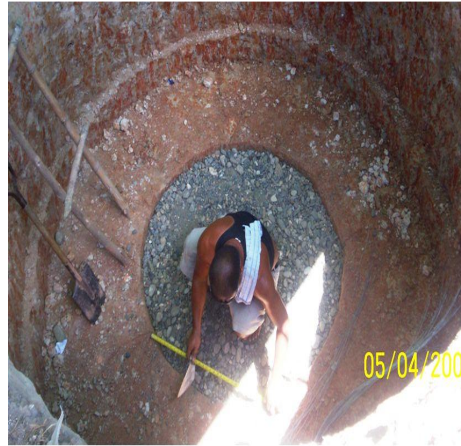
Gravel base course for the base
