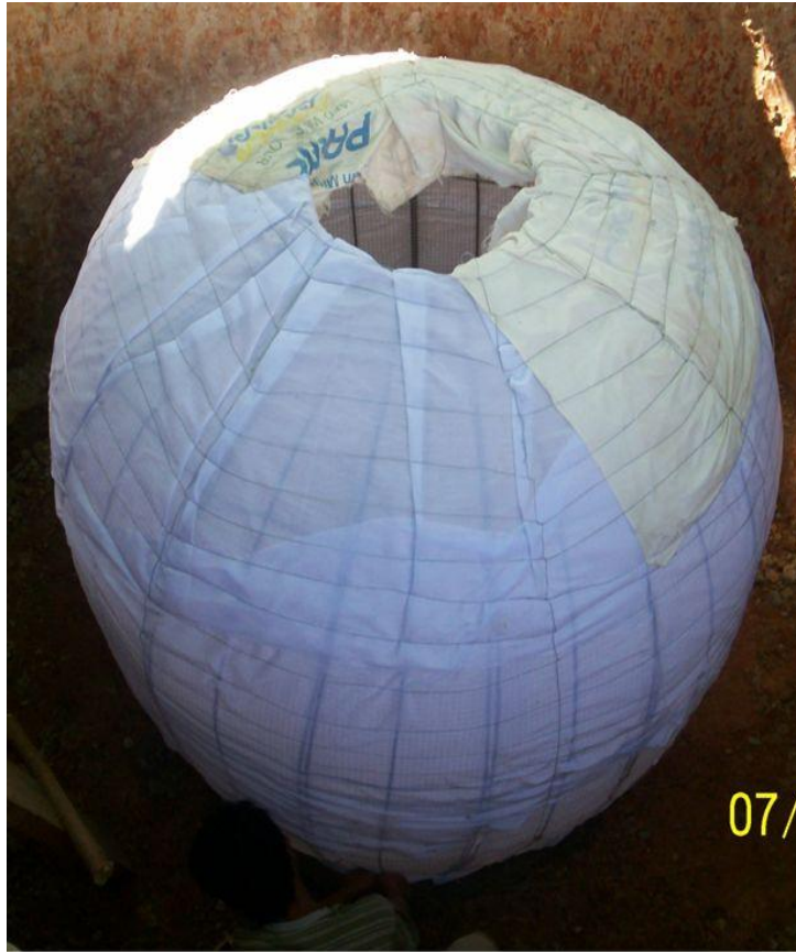
The digester mold wrapped in cloth and standing on the fresh-cast base
