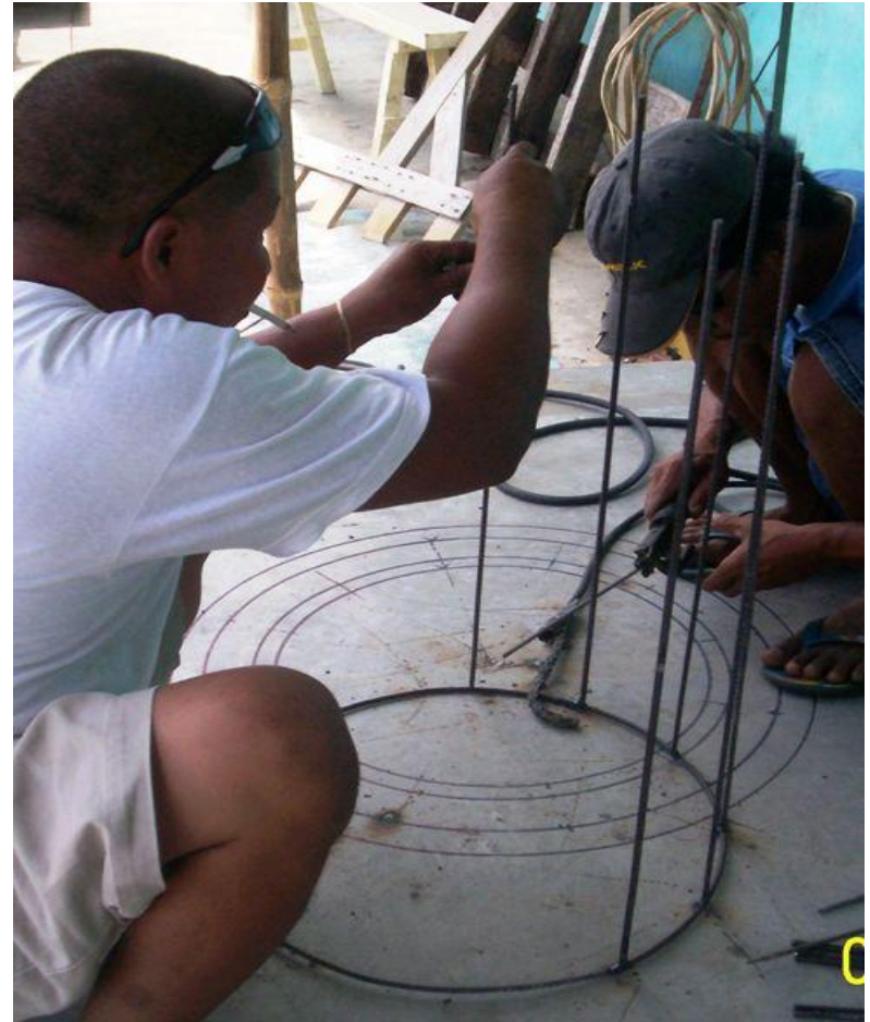
Walling-in culvert mold welding
