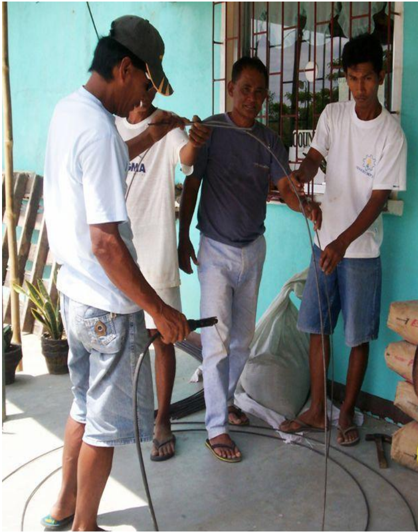
Welding the molds
