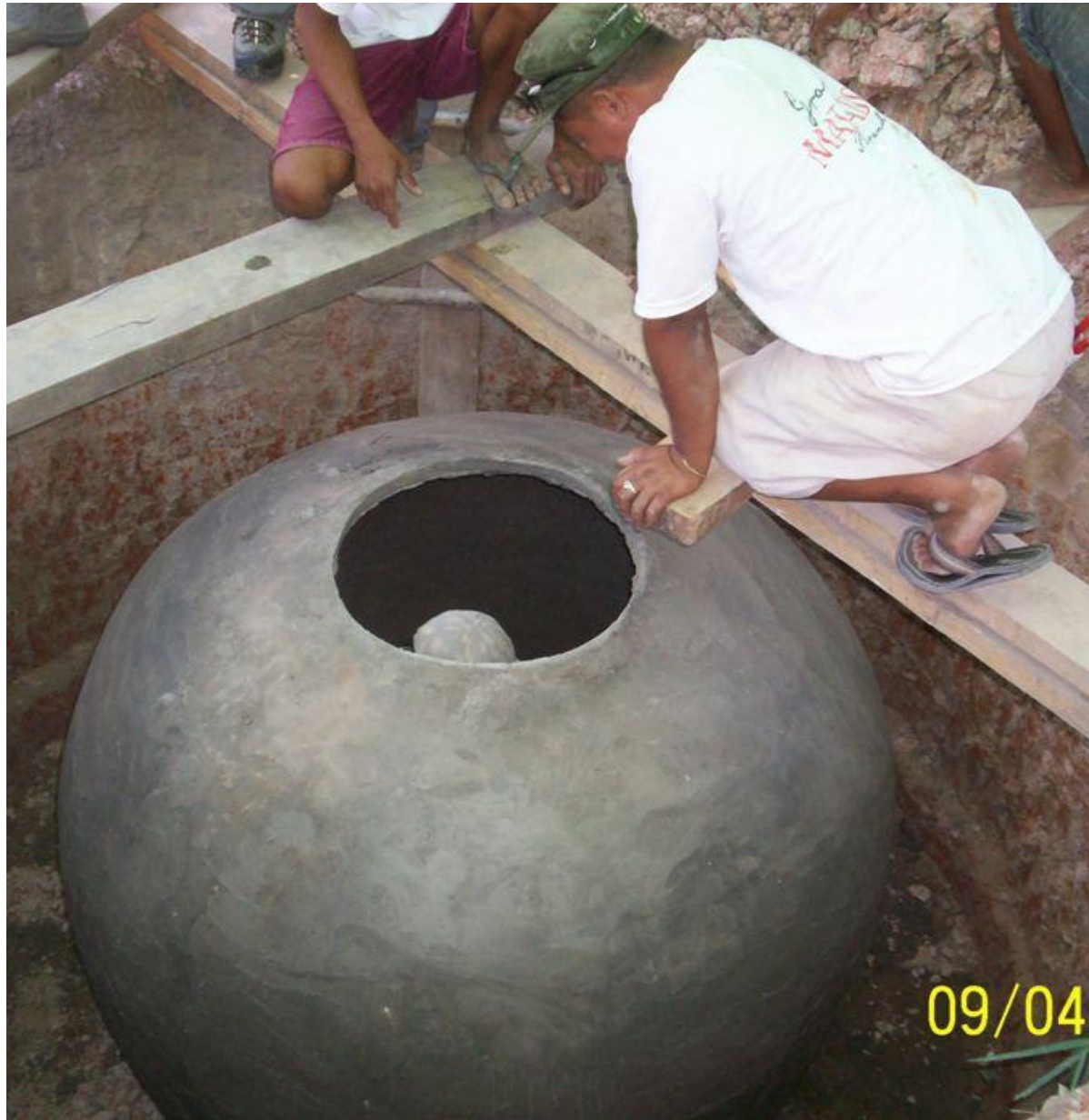
The digester is de-molded and finished inside.
