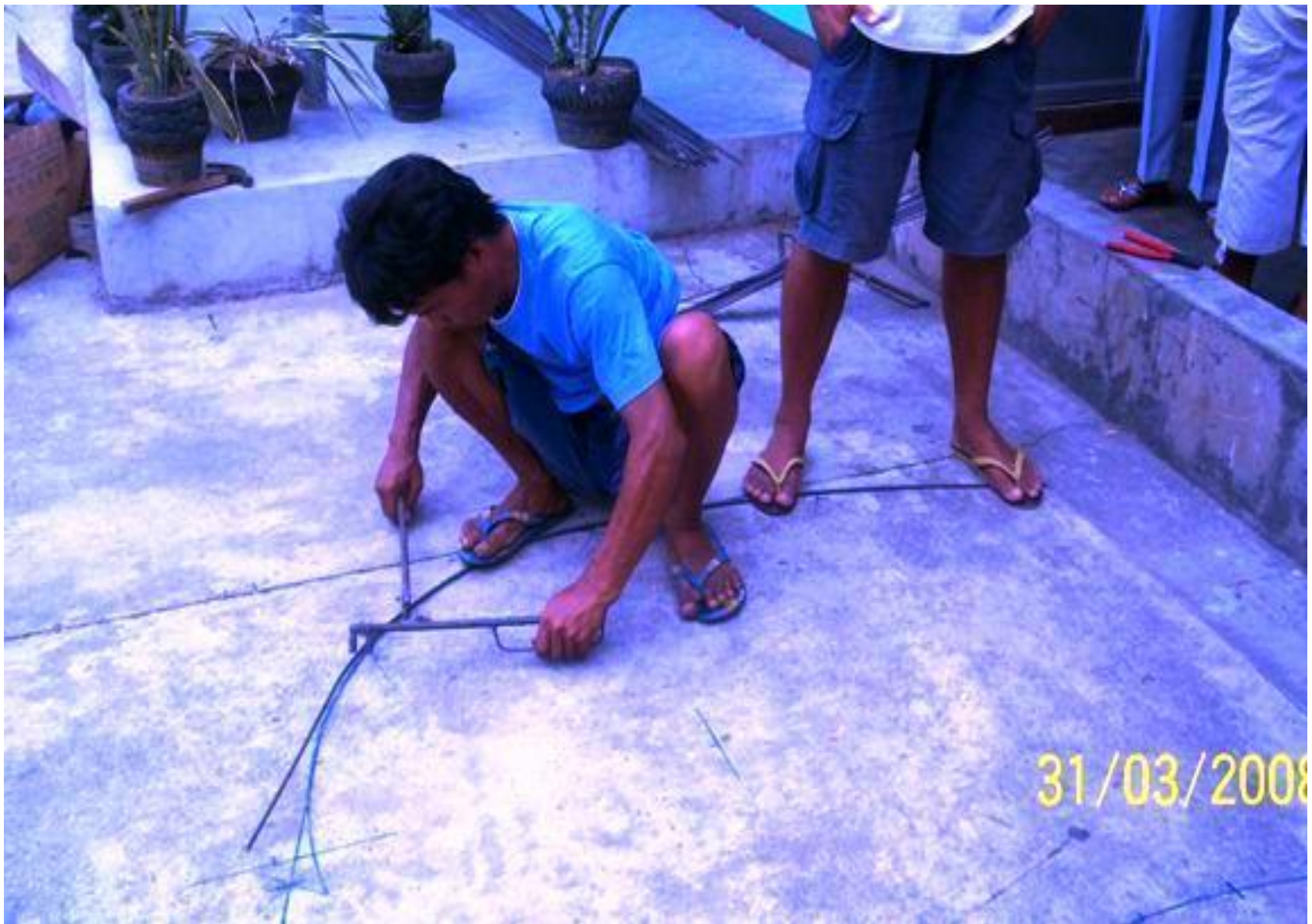
Bending the mold rebars
