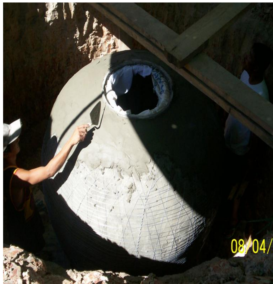
After the horizontal wiring is laid, a finishing mortar coat.
