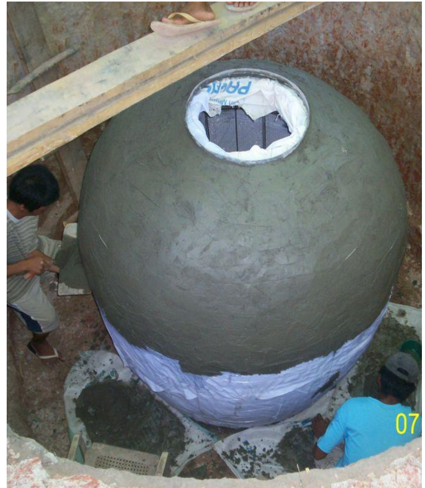
First mortar coating of the digester.
