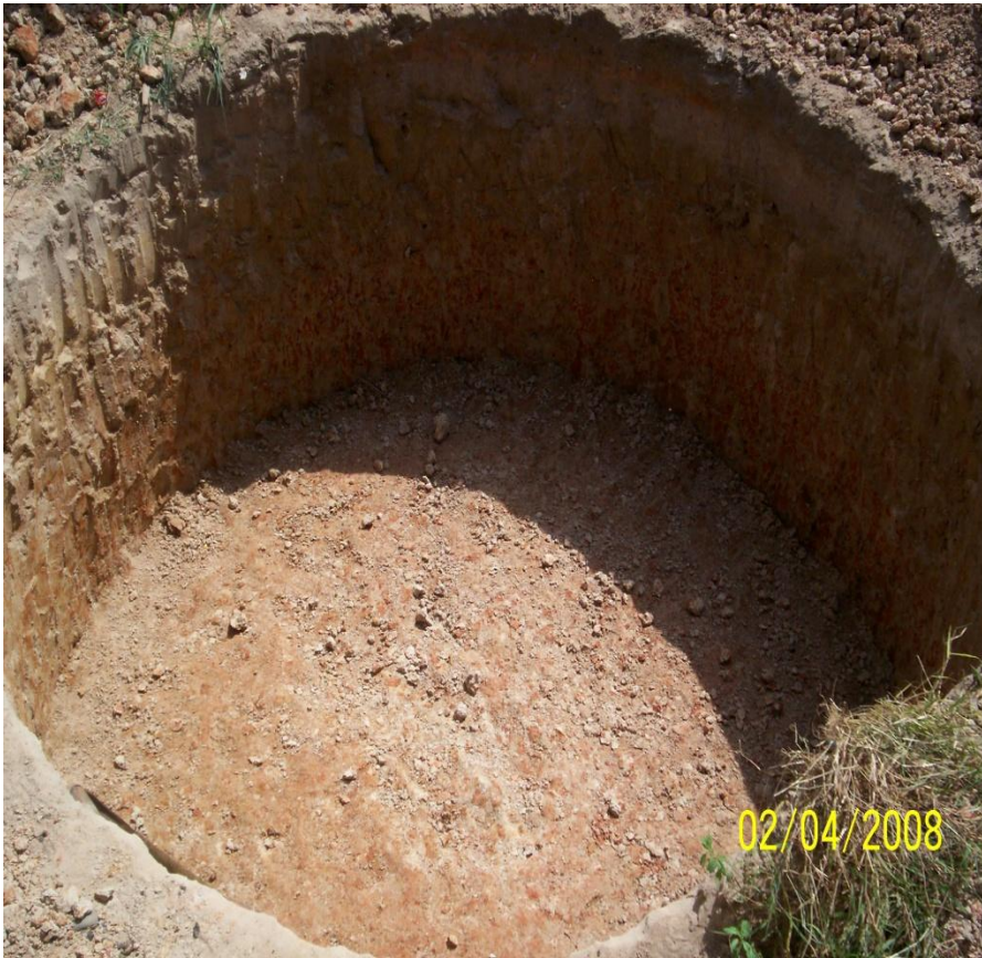
Meanwhile, the hole for the biogas digester is dug.
