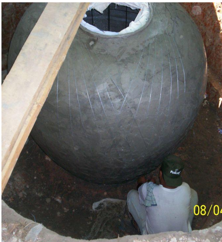
Vertical wires reinforcement for the digester
