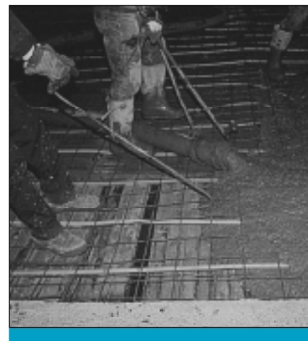
Fig. 3. Concrete is placed over tubing for a radiant floor.
