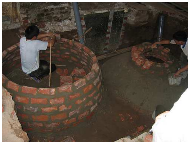
Figure 2. Construction of fixed dome household biogas plants for animal manure, which have toilets connected as well (near Hanoi, Vietnam). (source: F. Klingel, 2008). 4
