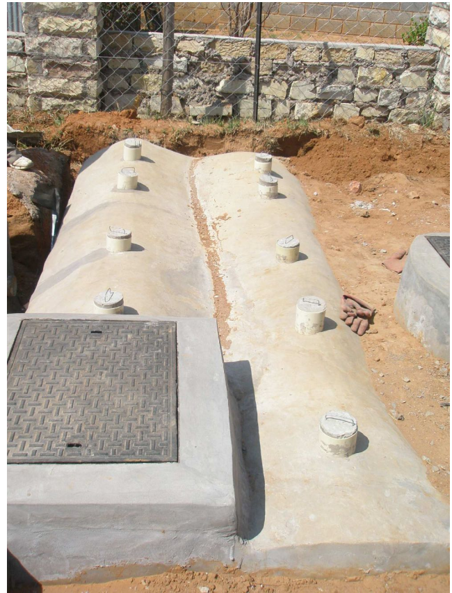
Figure 10: TED-BORDA Anaerobic Baffled Reactor in Maseru, Lesotho, 2009 (source: TED)
