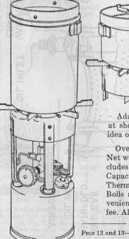
maximum output was required on the least weight and least space. It telescopes into two bayonet lock utensils in which the entire stove is packed.
