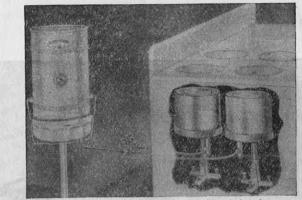
FIG. 14.—Victor range oil burner installed in stove. The illustration shows a two burner unit of the vaporizing type similar as shown on page 103.
