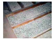
Photo - Attic Containing Vermiculite Insulation -
