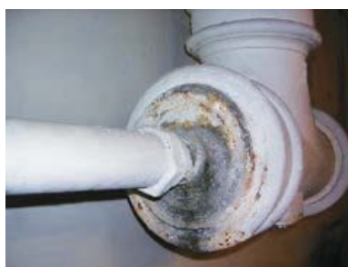
Figure 30 Amosite and chrysotile packing on waste pipes
