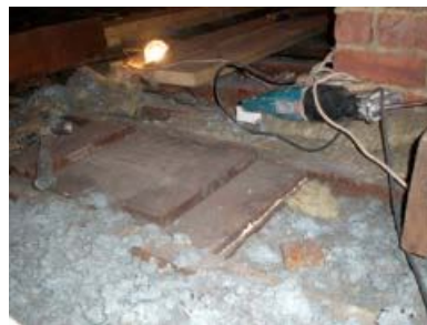
Figure 6 Loose asbestos used as loft insulation
