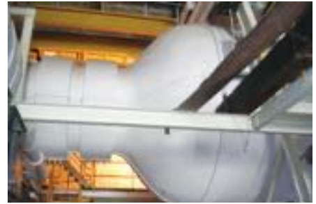
Figure 51 Vessel clad in amosite insulation
