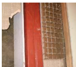
Figure 21 AIB column fire protection in CLASP building
