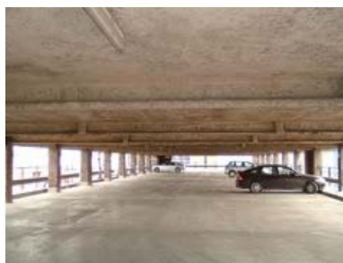
Figure 7 Sprayed limpet on car park roof
