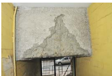
Figure 8 Sprayed coating on building passageway
