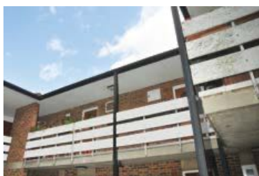
Figure 18 AIB exterior panel on open walkway
