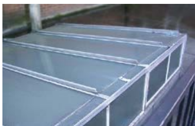
Figure 31 Chrysotile string on skylights
