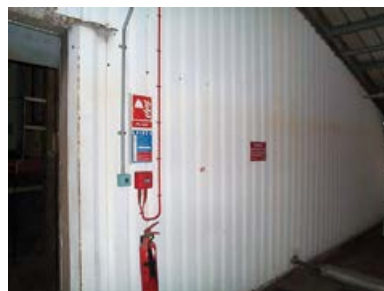
Figure 38 Chrysotile/bitumen coating under metal cladding
