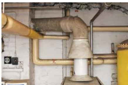
Figure 34 Asbestos cement boiler flue
