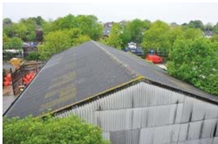
Figure 32 Asbestos cement roof and cladding
