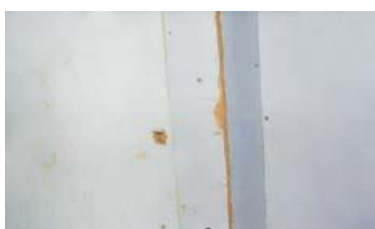
Figure 24 Chrysotile paper on fibreboard boxing
