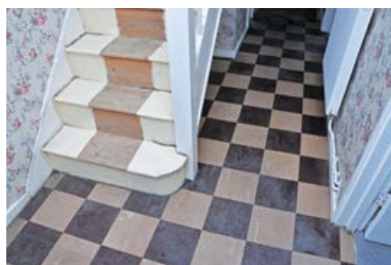
Figure 39 Asbestos-containing vinyl floor tiles
