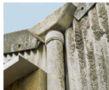
Figure 35 Asbestos cement downpipe
