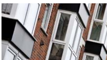
Figure 16 AIB exterior painted panel
