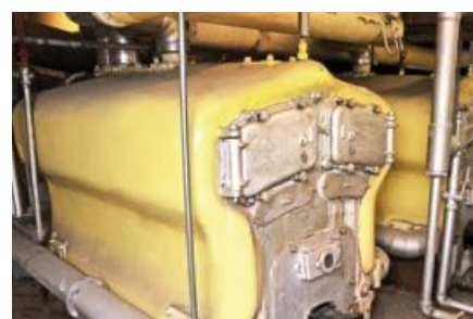
Figure 13 Amosite lagged boiler with hard plastic coating
