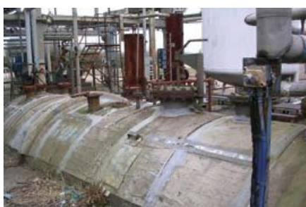
Figure 12 Lagging on large petrochemical vessel
