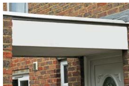
Figure 15 AIB panel in porch
