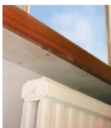
Figure 20 AIB panel between radiator and window
