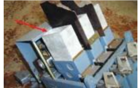
Figure 49 Electrical switchgear with asbestos flash protection
