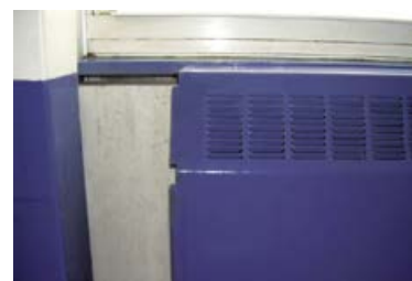
Figure 19 AIB behind school radiator unit
