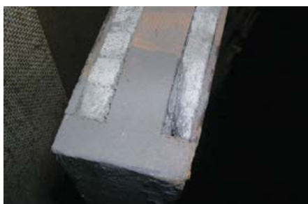
Figure 14 Asbestos panels inside fire door
