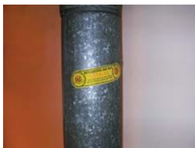
Figure 43 Metal clad gas flue containing chrysotile lining
