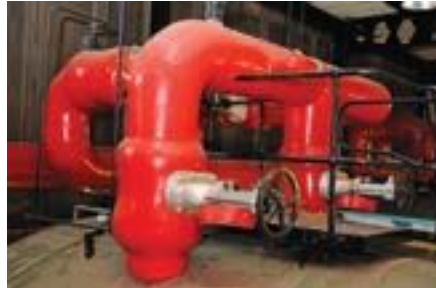
Figure 48 Asbestos-insulated supply pipes
