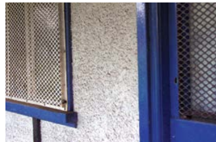
Figure 33 Chrysotile pebble-dash exterior wall coating
