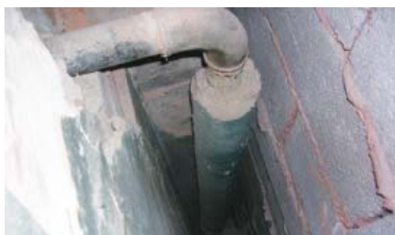
Figure 9 Lagged pipe in wall cavity
