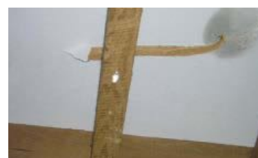
Figure 25 Chrysotile paper on strawboard ceiling panels
