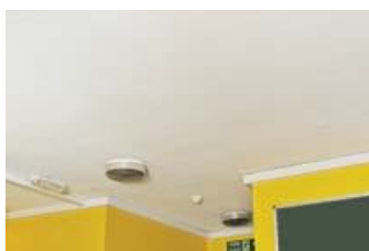
Figure 36 Asbestos textured coating on ceiling
