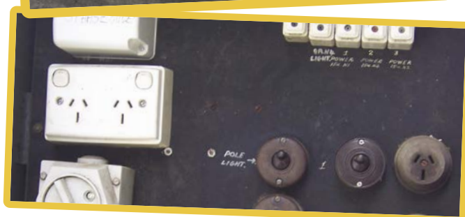
Zelemite backing board to an external switchboard
