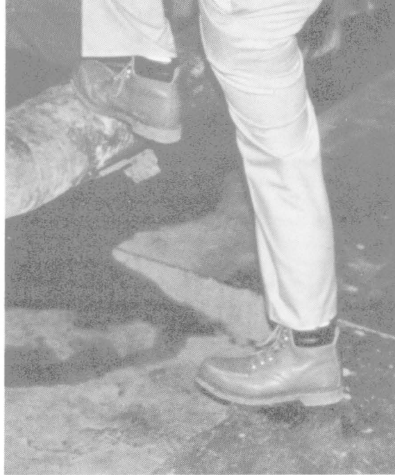
Routine maintenance activities can cause disturbance of ACM if workers are not properly trained in operations and maintenance procedures. Here, a worker carelessly contacts ACM, possibly damaging it.
