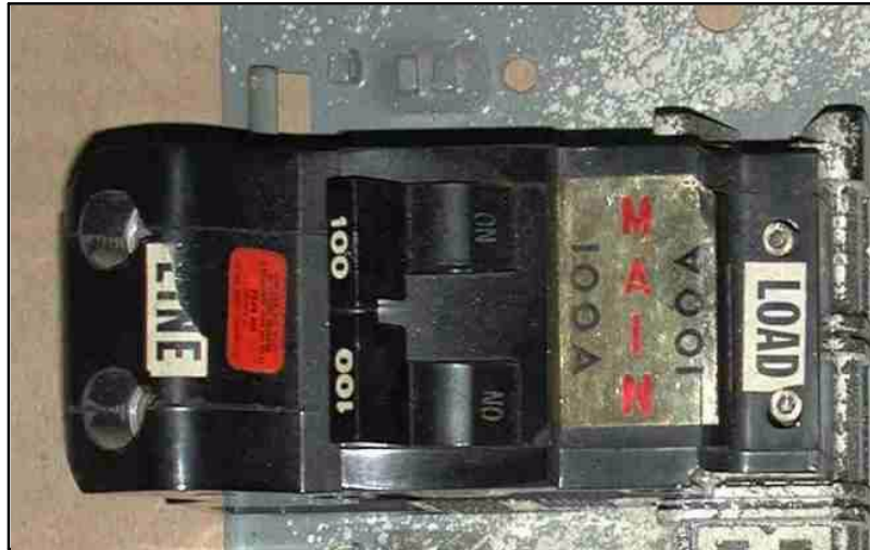
FIGURE 6 - FPE 100-AMP MAIN BREAKER CONNECTS TO THE BUSBARS THROUGH THE PLATE & POST CONFIGURATION, USING ONE SOCKET-HEAD 8-32 SCREW FOR EACH POLE TO ATTACH TO ITS CONTACT PLATE. (The heads of the 8-32 clamping screws are seen at right, above and below the "LOAD" label.)
