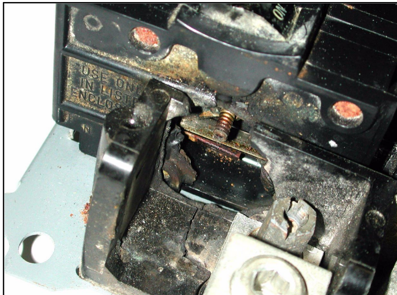
FIGURE 9 - VIEW DOWN TOWARD UPPER RIGHT OF PANEL SHOWN IN FIG. 8. THIS FPE STAB-LOK® TWO-POLE 30-AMP BREAKER FED THE CLOTHES DRYER.
