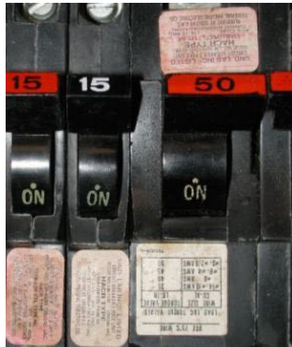
FIGURE 12 - FPE STAB-LOK ® BREAKERS WITH WHITE DOT ON TOGGLE (ABOVE “ON”) AND PINK LABEL
