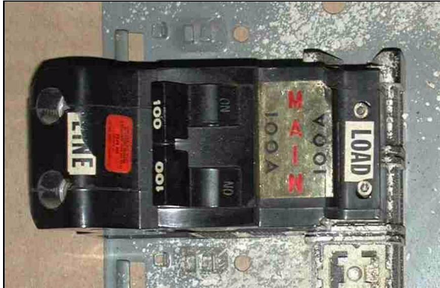
FIGURE 6 - FPE 100-AMP MAIN BREAKER CONNECTS TO THE BUSBARS THROUGH THE PLATE & POST CONFIGURATION, USING ONE SOCKET-HEAD 8-32 SCREW FOR EACH POLE TO ATTACH TO ITS CONTACT PLATE.
