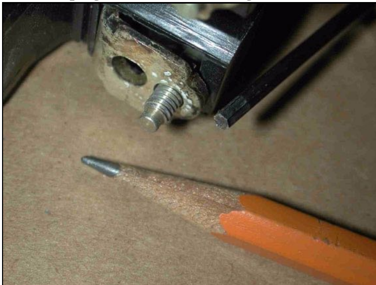
FIGURE 7 - ONE LOAD-SIDE CONTACT AND ITS 8-32 CLAMPING SCREW, ON THE FPE 100-AMP MAIN BREAKER OF FIG. 6. THE SCREW-HEAD TAKES A 3/32" ALLEN WRENCH, WHICH IS ONLY SLIGHTLY LARGER THAN THE LEAD OF THE PENCIL.
