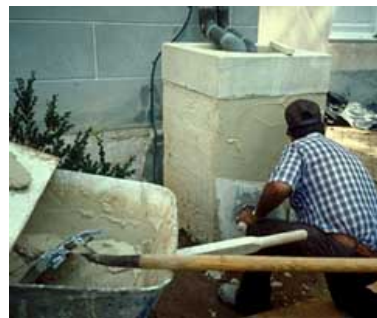
The deteriorated surface of this catch basin is being re-stuccoed. Photo: NPS files.
