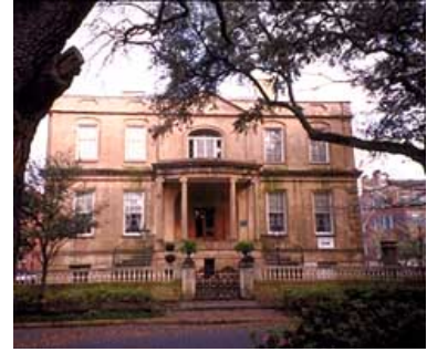
The stucco on the early-19th century Richardson-Owens-Thomas House in Savannah, Georgia, is a type of natural cement. Photo: NPS files.
