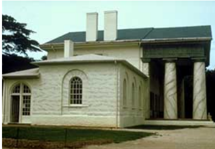
The stucco finish on Arlington House, Arlington, Virginia, was marbleized in the 1850s, approximately 30 years after it was built. Photo: NPS files.
