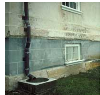
The damage to this stucco appears to be caused by moisture infiltration. Photo: NPS files.
