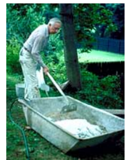
The dry materials must be mixed thoroughly before adding water to make the stucco. Photo: NPS files.
