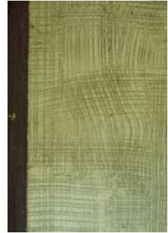
The final finish coat will be applied to this scratch coat. Photo: NPS files.
