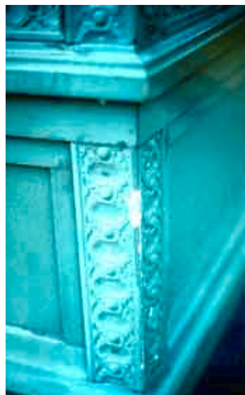
Substitute materials need to be located with care to avoid damage. The fiberglass column base has chipped, whereas the historic cast iron would have remained sound. Photo: NPS files.
