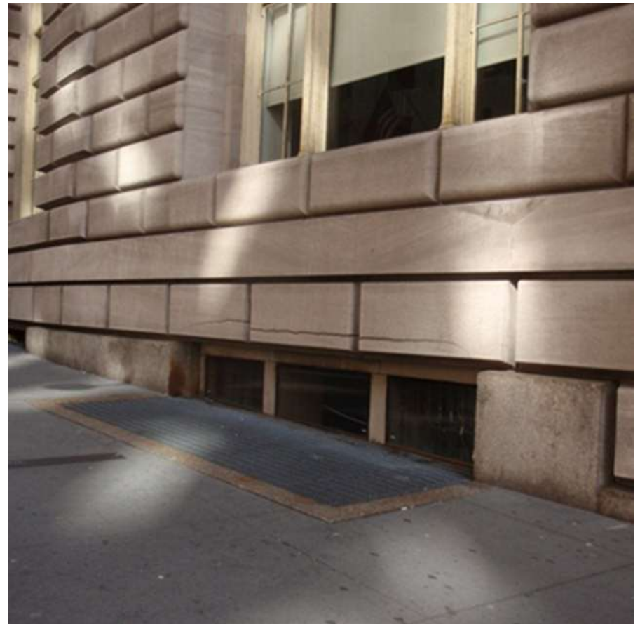
Horizontal Crack
