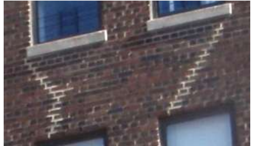
Repaired Stepped Crack
