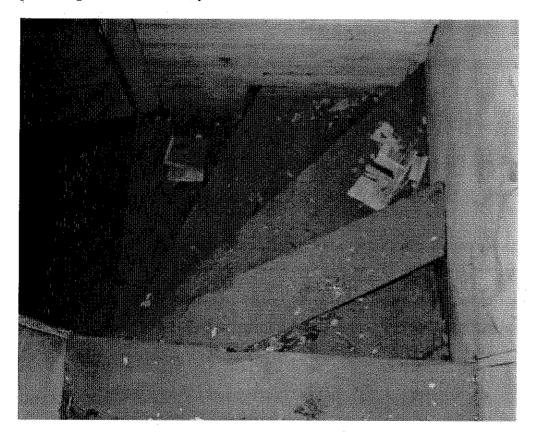
Figure 28: Some of the stair treads, particularly in the winding section, are broken.
