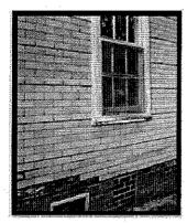
Rolled asphalt brick siding was made possible through the introduction of heated rollers that pressed patterns into the surface.
