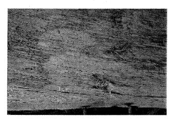
Figure 10: The round "log" joist on the left has evidence of powderpost beetle damage—a scattered pattern of tiny holes, about 1/16 inch in diameter. The beetle primarily attacks the sapwood of wood that has not had time to dry completely. Damage from powderpost beetles can result in the sapwood (outer 2 inches or so of each log) being largely hollow, reducing the structural capacity of the member from that of the profile that appears to be represented.
