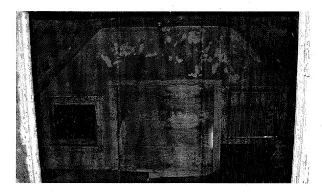
Figure 25: The second story (or attic) consists of two large rooms shaped by the roofline, knee-walls, and a narrow ceiling. Beneath twentieth century plaster on expanded metal lath, the original wall treatment of horizontal bands of beaded interior sheathing appears to be intact.
