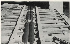
G-E Fiberduct in sleeper type floor construction
