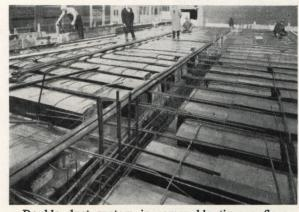
Double duct system in removable tin-pan floor construction
