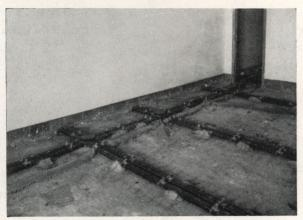
Double duct system showing Prelokaylets installed in factory on two-foot centers
