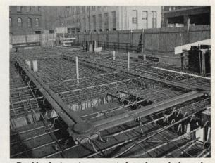
Double duct system mounted on formed channel steel supports
