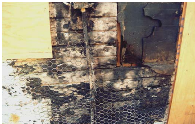
Fig. 9. Extensive burning of the exterior of a house which became electrified due electrical contact with the metal plastering mesh (Photo: Al Graps).
