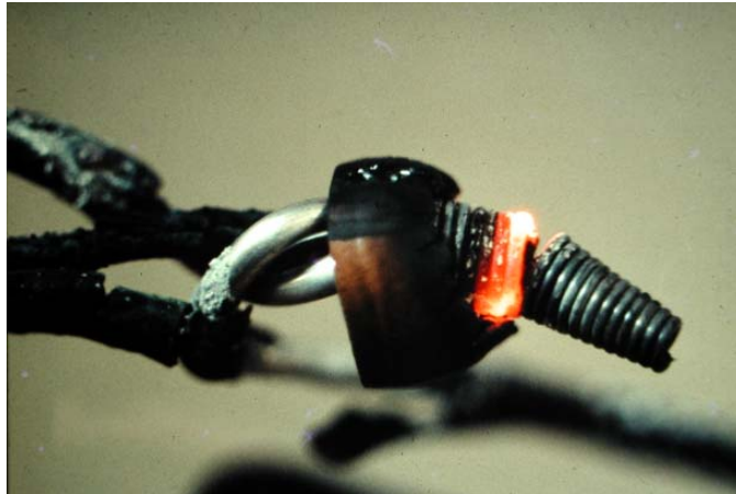
Fig. 1. Failure of a twist-on connector due to insufficient tightening; note that the plastic outer insulator of the connector has nearly melted away and only a small shoulder remains, allowing the internal helical spring to be exposed (Photo: Jesse Aronstein).
