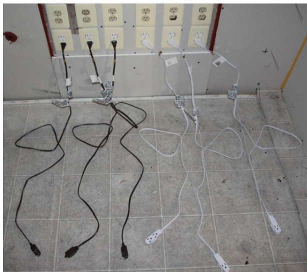
Figure 3-4. Location and arrangement of extension cords in compartment.
