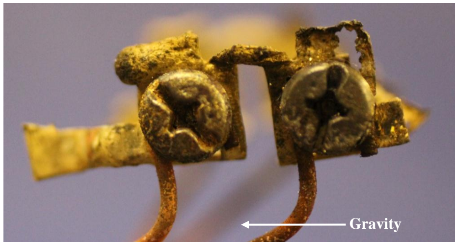
Figure 3-39. Photograph of melted brass receptacle contact showing round globule and effects of gravity (LEV354, non-energized).
