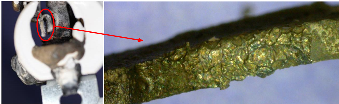
Figure 4-17. Small divots (and localized round depressions) on a grounding strap from a neutral to ground arc during receptacle failure (LEV008).
