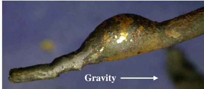
Figure 3-48. Photograph of melted copper wiring showing irregular end and effects of gravity from a non-energized PVC receptacle (PSE386).
