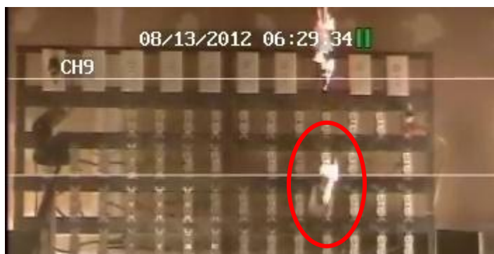
Figure 2-48. Flaming faceplate drops to ground (PSE166).
