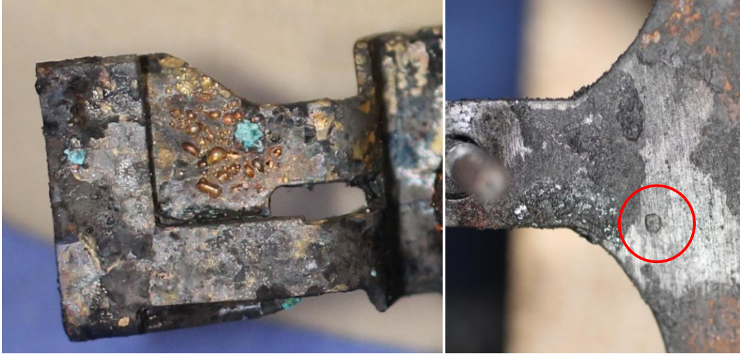
Figure 4-26. Surface pitting on brass contacts from PSE358 (left) and corresponding arcing damage on faceplate from PSE323 (right).
