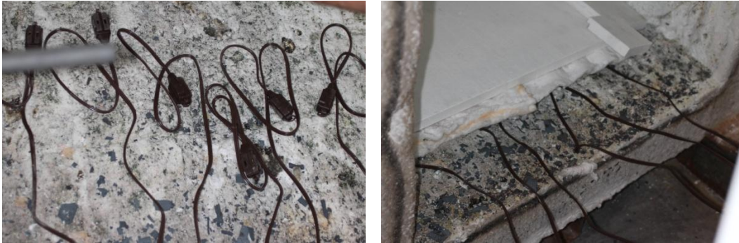
Figure 3-8. Location and arrangement of extension cords in furnace (left) and insulation placement (right).
