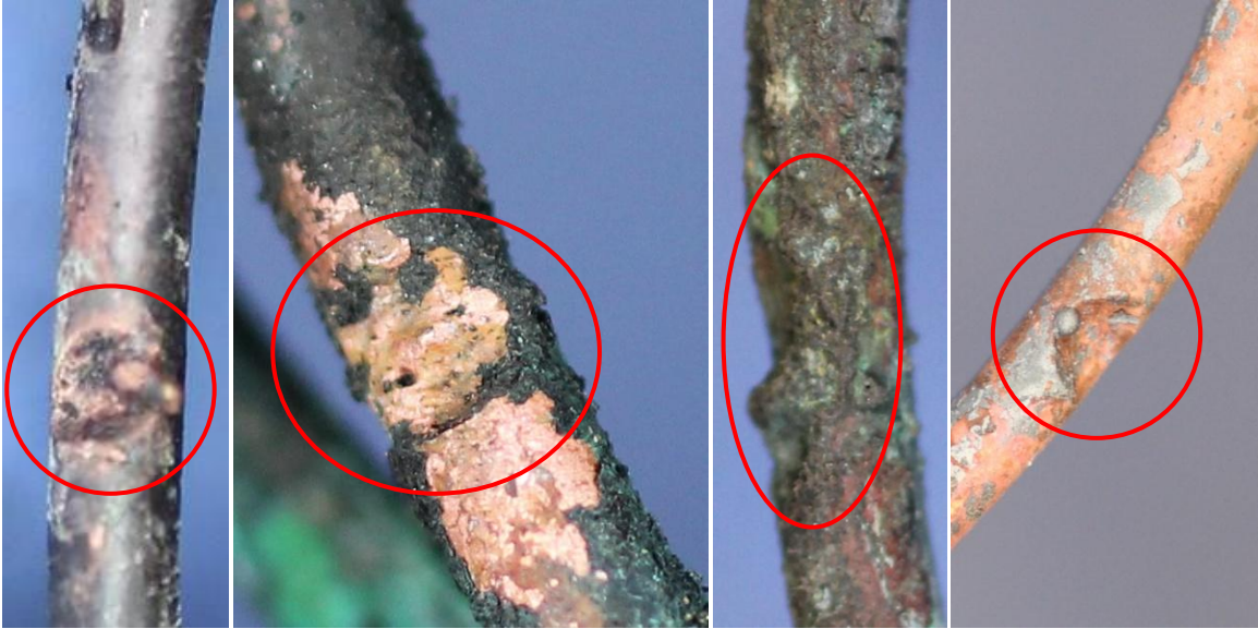
Figure 3-57. Arcing evidence on wiring from four thermostet receptacles (From left to right: B010, D035, E078, and E083).
