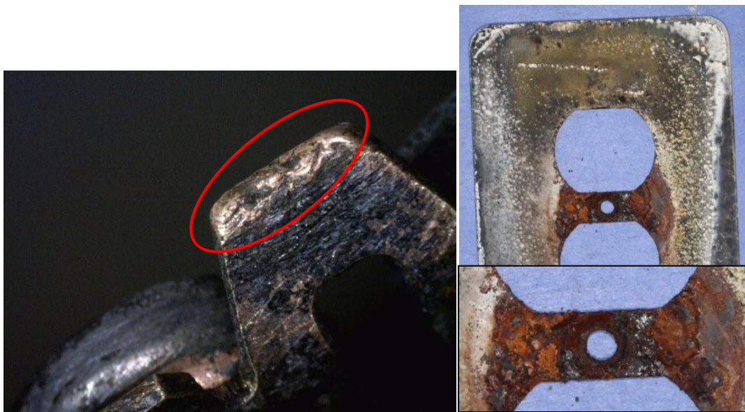
Figure 3-56. Photos of possible arcing damage on break off tab of energized PVC receptacle (PSE251, left) and rusted steel faceplate (right).
