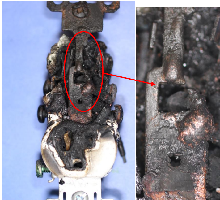
Figure 4-3. Localized point of contact without a sharp line of demarcation (PSE 285).
