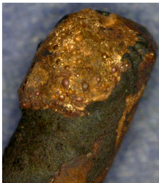
Figure 4-19. Solid copper conductor with blisters on the surface (PSE385).
