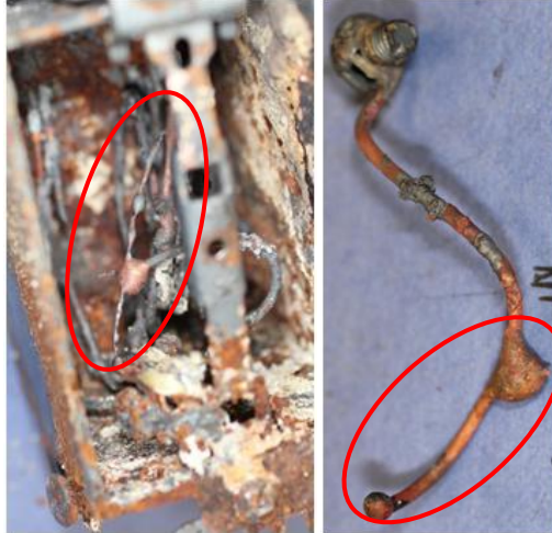
Figure 3-53. Photographs of melted copper wiring from energized polypropylene receptacles LEV398 (left) and LEV400 (right).
