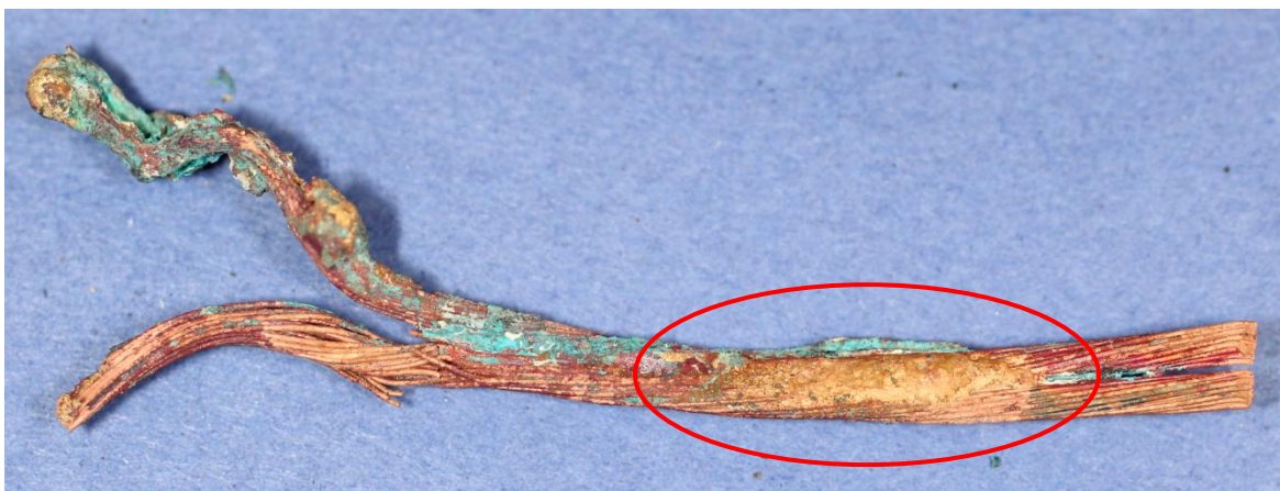
Figure 4-1. Corresponding damage on opposing conductor(s) for receptacle with melting (LEV397).
