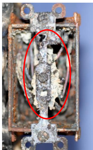
Figure 3-17. Photograph of totally consumed PVC receptacle with copper melting (PSE385) showing remaining char.
