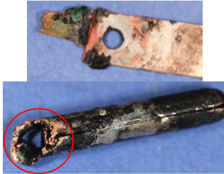
Figure 2-77. Arcing damage at back of ground pin (bottom); hot blade (top) from plug in receptacle LEV286.
