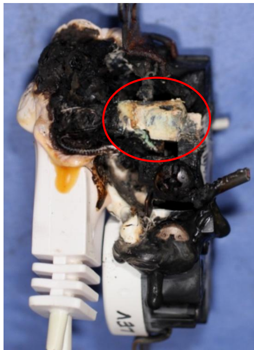
Figure 2-78. White residue (corrosion) at plug/receptacle connection (LEV060).
