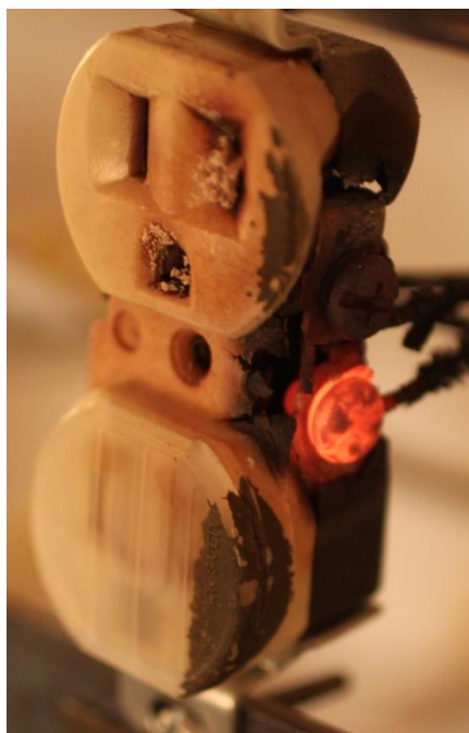
Figure 2-39. Thermoset receptacle with overall glow at ¼ turn loose connection (E010).
