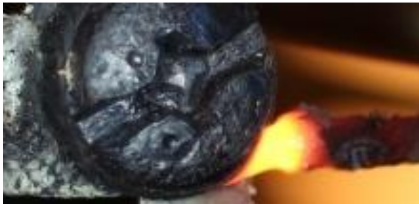
Figure 2-42. Necking of conductor at glow spot on receptacle LEV277.
