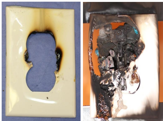
Figure 3-22. Photographs of typical faceplate damage from overheating connections: LEV171 (left) and LEV269 (right).
