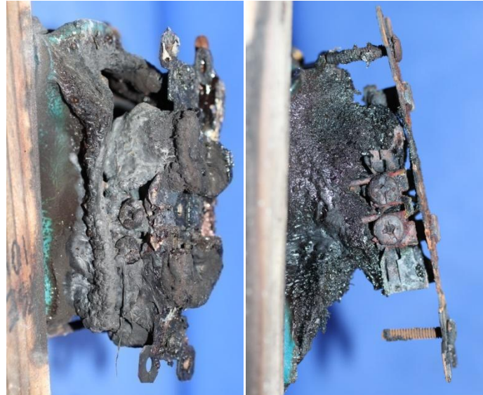
Figure 3-10. Thermal damage to PVC receptacles: mostly consumed (PSE101, left) and totally consumed (PSE137, right).
