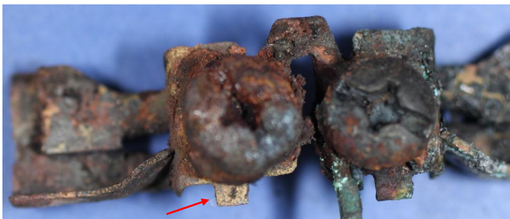
Figure 3-100. Photograph of internal plug contacts thinned by oxidation and overheating from PVC receptacle (PSE021).
