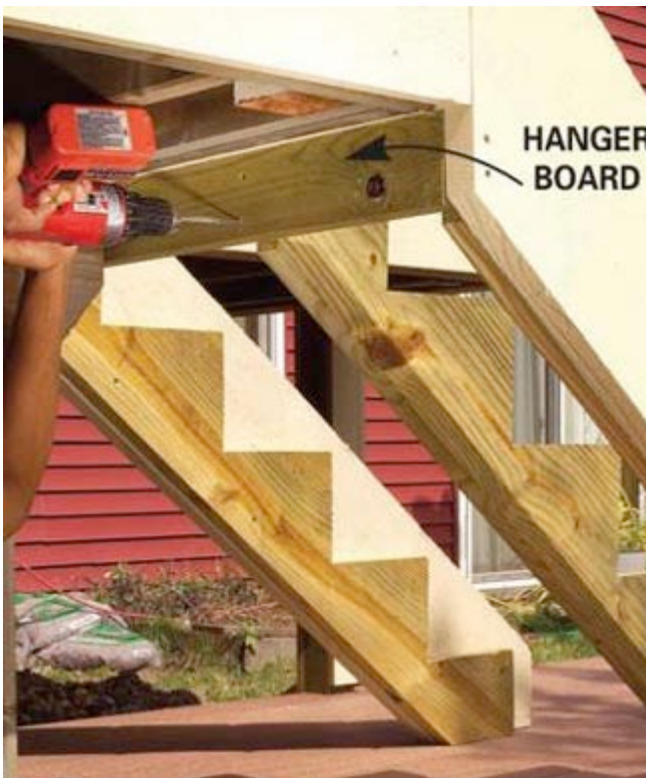
Stringers screwed to hanger board.
