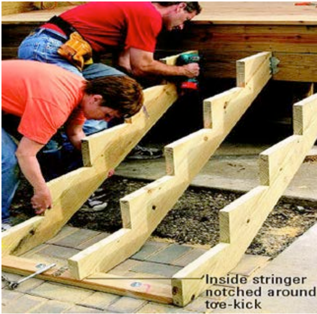
Stringer held firm at bottom by toe kicker being bolted at the bottom and brackets screw fixed to deck side face.
