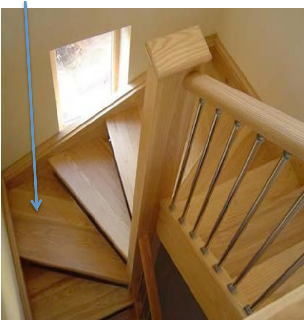
Dog Legged with Quarter spaced Landing and Winders
