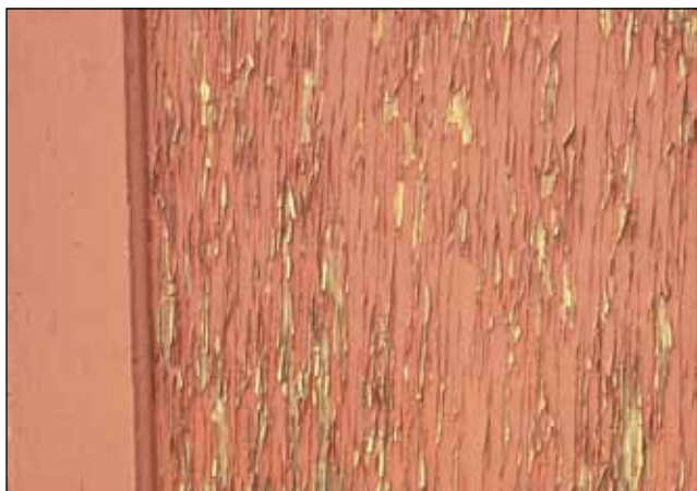
Figure 16-9. Early paint failure on plywood caused by penetration of moisture into surface face-checks.
