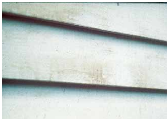
Figure 16–25. High moisture content of wood can cause diffuse extractives bleed, particularly if a stain-blocking primer is not used.
