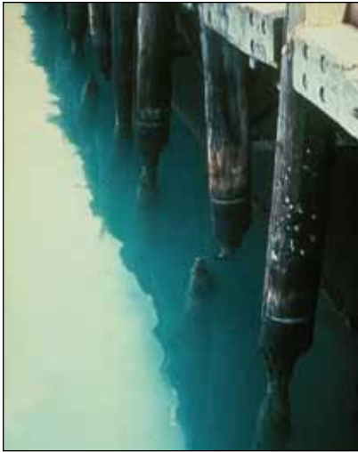
Figure 14-11. Limnoria damage to piling.
