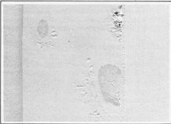
Figure 6. Brown discoloration of paint from resin exudation from a knot.
