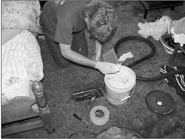
(left) After the duct is cleaned, fibred tape and mastic are used to air seal. A paint brush is the easiest ways to apply the mastic to the duct. (right) The end of the blow tube should be cut at an angle to help the tube slide over the existing insulation and past any obstructions in the cavity.
