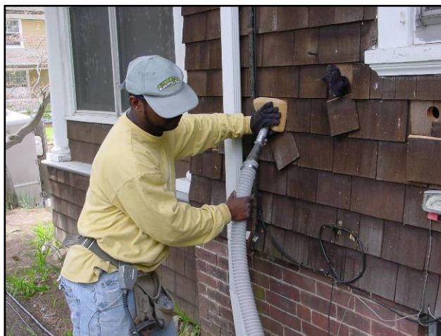
The one-hole method using a tube long enough to reach to the furthest corner of the cavity is the best way to dense pack walls
