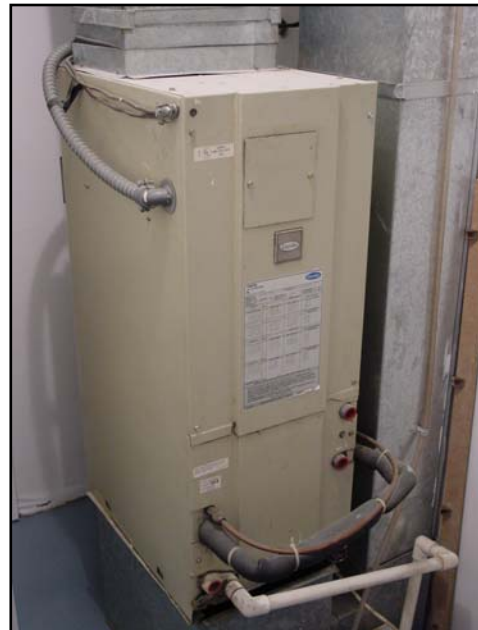
Carrier residential air source heat pump
