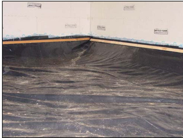
Ground cover sealed to foundation walls
