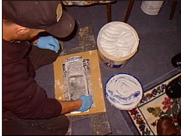
Sealing a register boot with duct mastic
