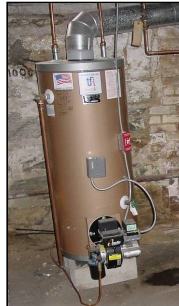
Oil-fired water heaters are not common
