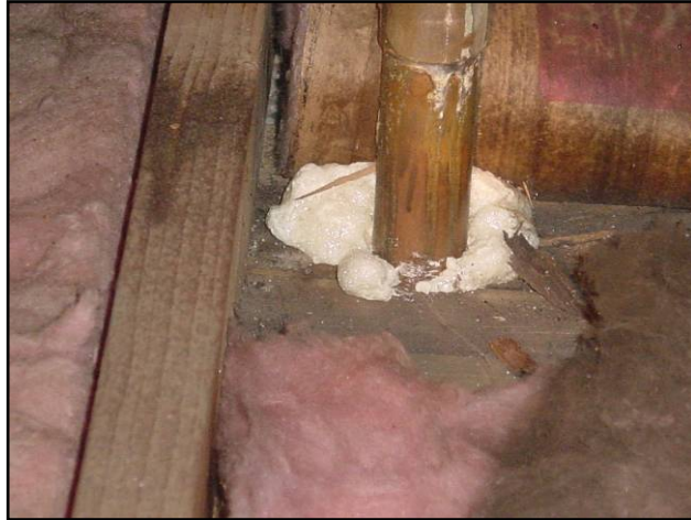
Plumbing stack sealed with foam
