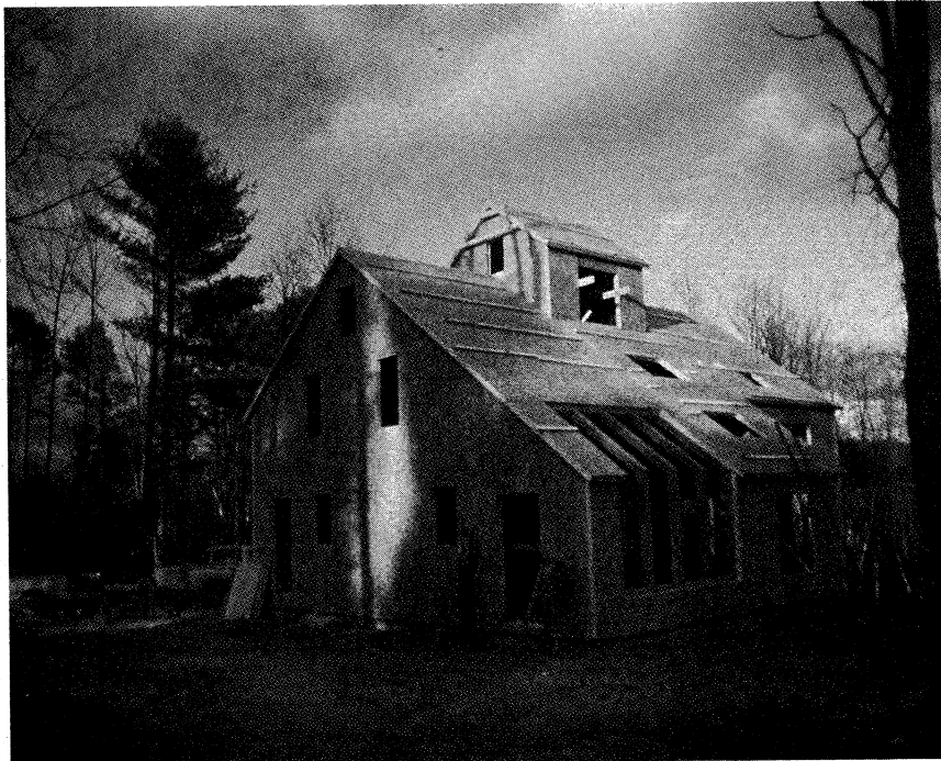
The old-fashioned way: Benson Woodworking Company in Alstead Center, N.H., builds heavy timber frames with plenty of hand chiseling, complex joints, and a precision fit. Benson has stress-skin panels made to specific thicknesses for custom homes.
