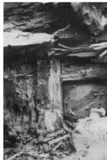
The west face of the house (above) was cut open in four spots, all revealing severe decay of the timber frame and adjoining wood. The southwest corner (below left) and center holes (below right) are shown close up.
