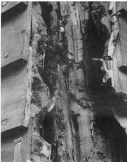
The west face of the house (above) was cut open in four spots, all revealing severe decay of the timber frame and adjoining wood. The southwest corner (below left) and center holes (below right) are shown close up.
