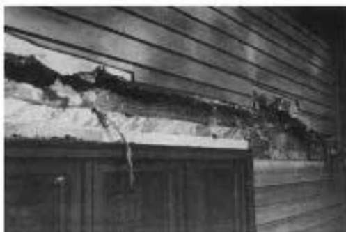
The beams were heavily checked on the inside (right) and rotting on the outside (left).
