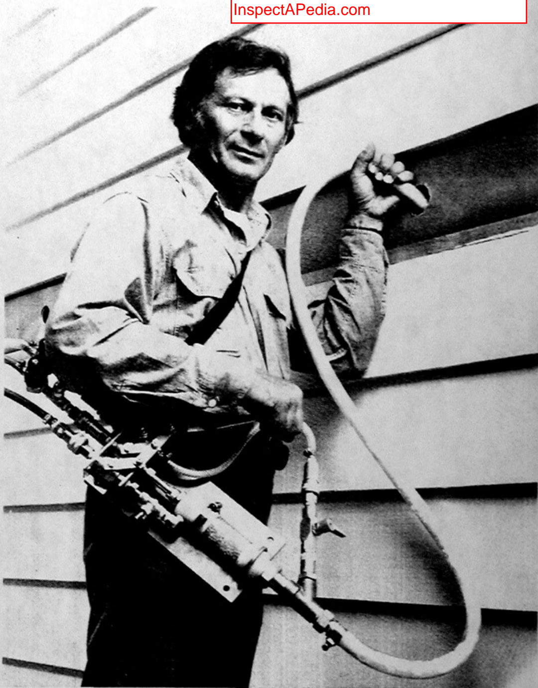
1: This new insulation made from ultra-lightweight cement combines high R-value, excellent fire resistance, and the ability to flow into nooks and crannies.
