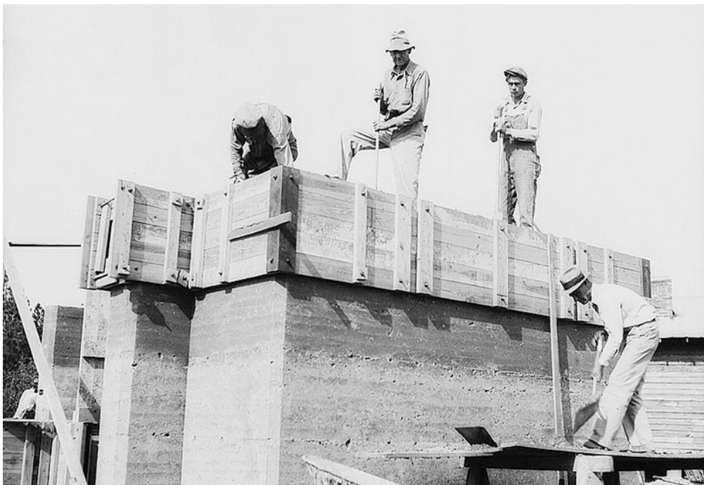
Figure 10. Workmen adding rammed earth layers to a wall at Gardendale (photographs from the Library of Congress, Prints and Photographs Division).
