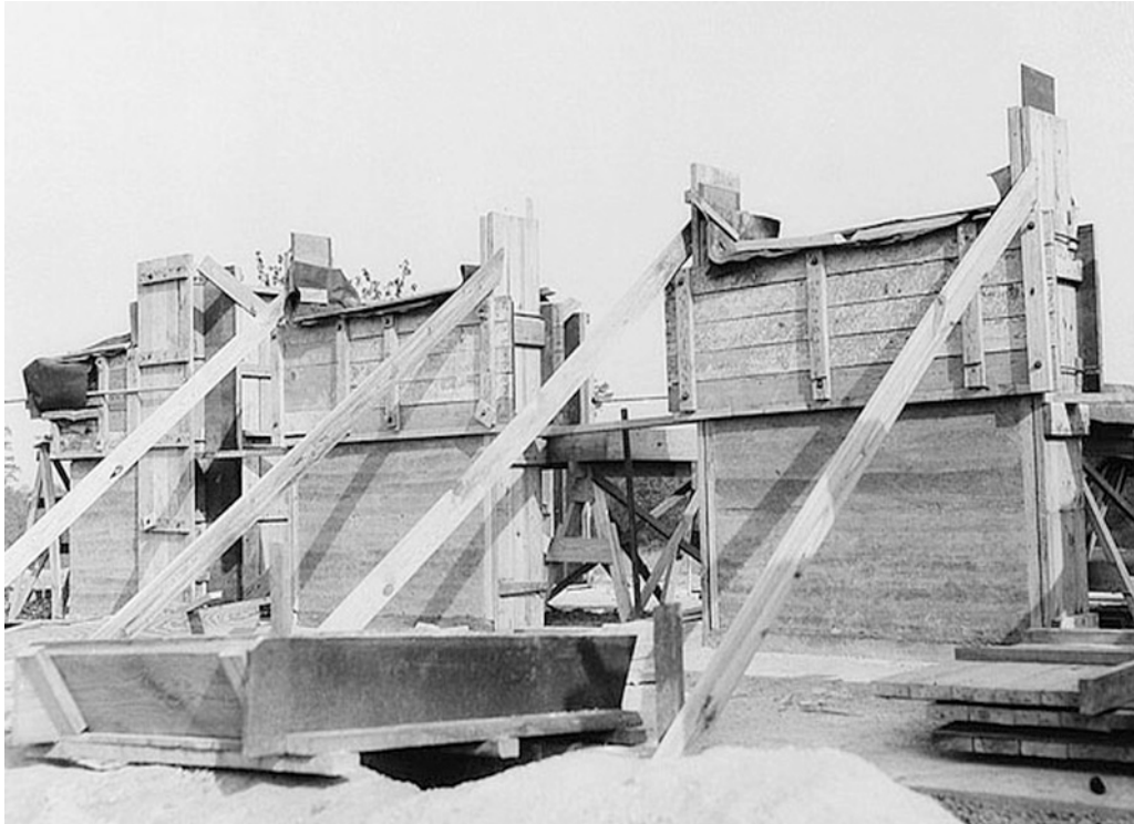
Figure 9. Erected shuttering for the rammed earth homes at Gardendale.
