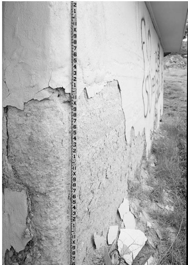
Figure 33. View of the deteriorating rammed earth wall at Cameron Valley ( photographs from the Library of Congress, Prints and Photographs Division, Historic American Buildings Survey ).
