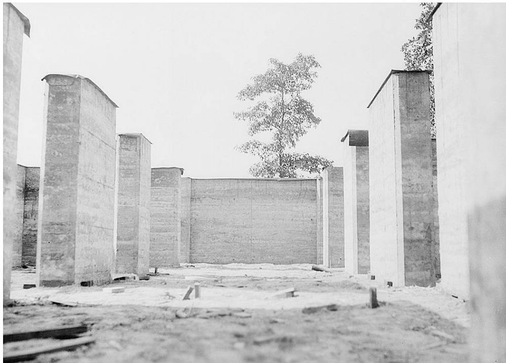
Figure 13. Completed rammed earth walls at Gardendale ( photograph from the Library of Congress, Prints and Photographs Division ).
