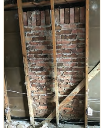
PHOTO 5 Backside of Brick. Now it gets interesting, especially if you have brick. You cut away and get rid of all the interior gypsum board and cavity insulation and your sheathing, leaving bare stud framing and naked exposed brick. When in doubt, throw it out.
