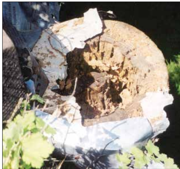
Figure 1.10—Damage to a bridge piling.
