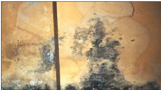
Figure 1.7—Close-up of the severely stained and discolored ceiling panels.
