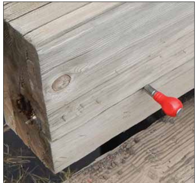
Figure 2.2—An awl is used to assess depth and presence of decay in a horizontal split.
