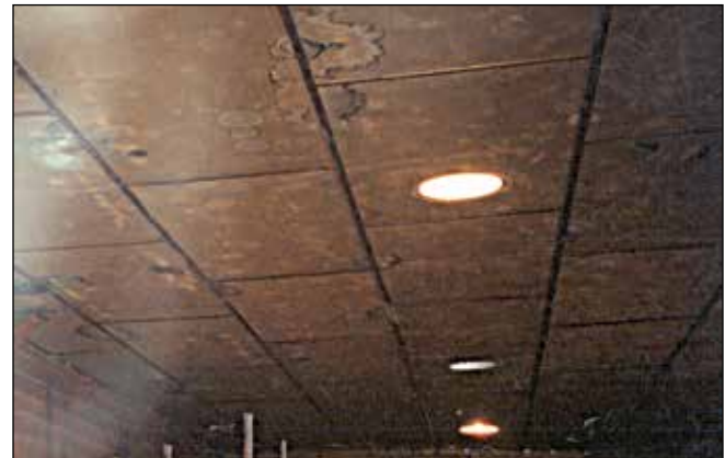
Figure 1.6—The ceiling panels were stained and discolored.
