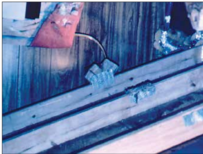
Figure 1.11—Metal plate connectors were cut and bent so that the webs could be removed. This should never be done.
