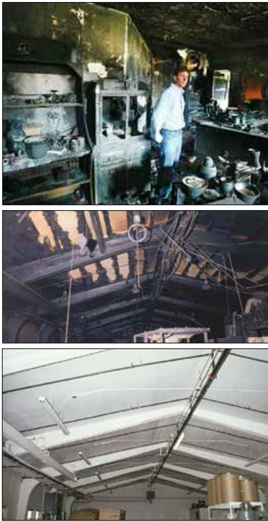
Figure 5.10—Post-fire inspection (top) of residence; post-fire (middle) and post-repair (bottom) of Building 2 at the Forest Products Laboratory. Top photo courtesy Montana Standard; www.mtstandard.com .
