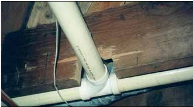
Figure 1.14—A floor joist was cut to make room for plumbing. This should never be done.
