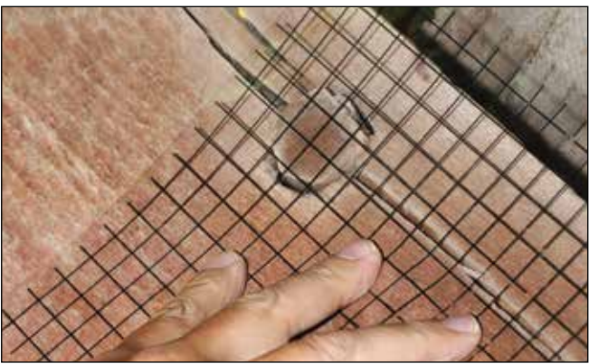
Figure 6.6—Example of using grid to establish the size of knot in bridge member. The measured knot in the example is 1-1/2 in.
