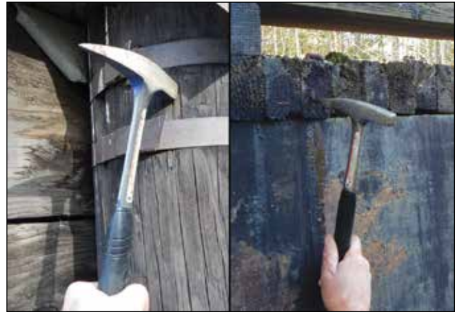
Figure 2.1—A hammer pick is an effective tool for initial assessments of timber bridge elements.
